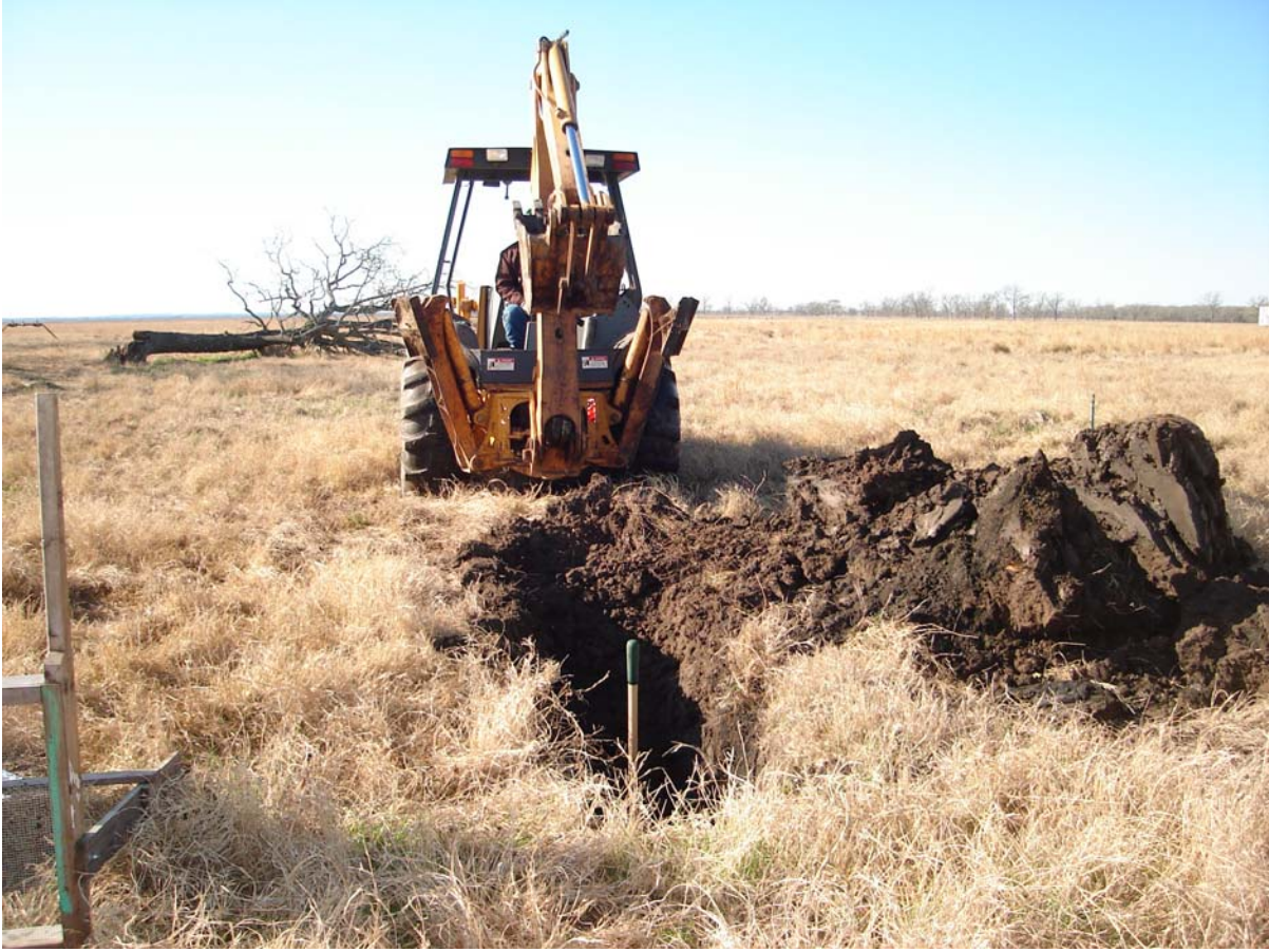
Figure 7. Backhoe Trench 2 (A-1 Well)
