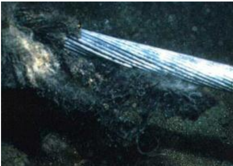
(c) Cable damage by trawl gears
