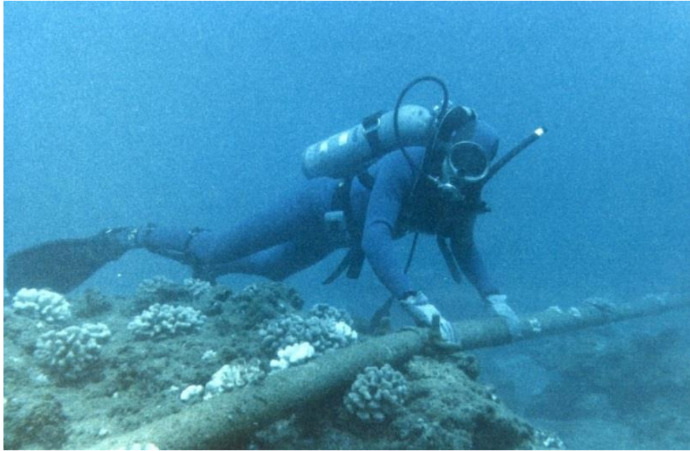
Fig. 1.2 An example of a submarine power cable inspection (Heimbuch, 2010)
