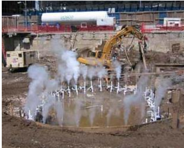
Figure 2.3 Ground freezing for sinking shafts (Moretrench, 2011)
