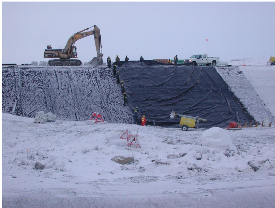
Figure 2.2 Construction of a frozen core dam (Nuna Logistics, 2014)
