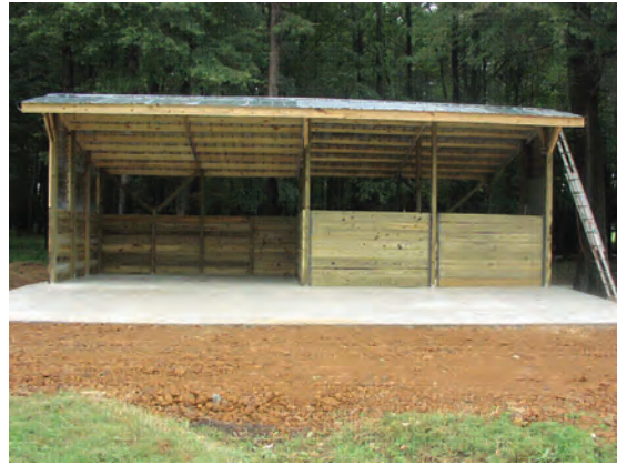
Proper composting barn
