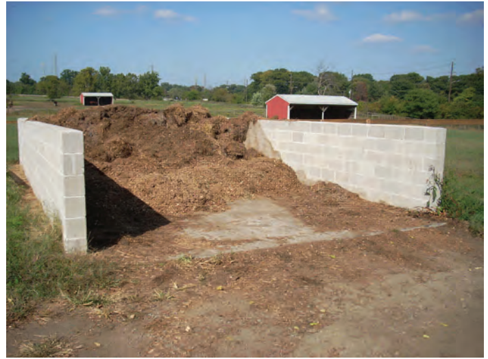
Manure storage area
