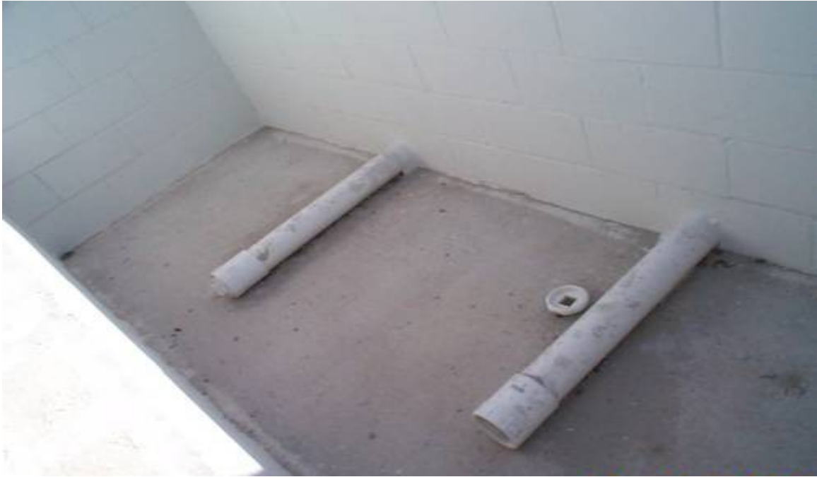
Figure A.3 Reservoir without water
