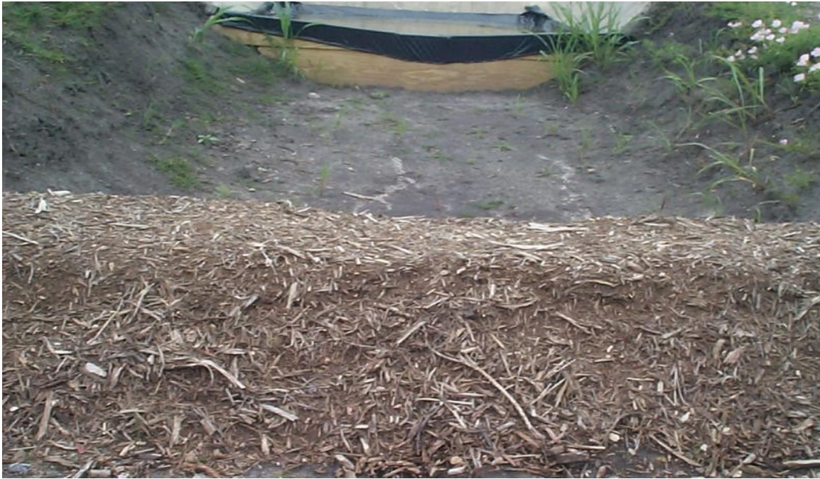
Figure 5.38 Yard waste compost berm before starting the structural testing.
