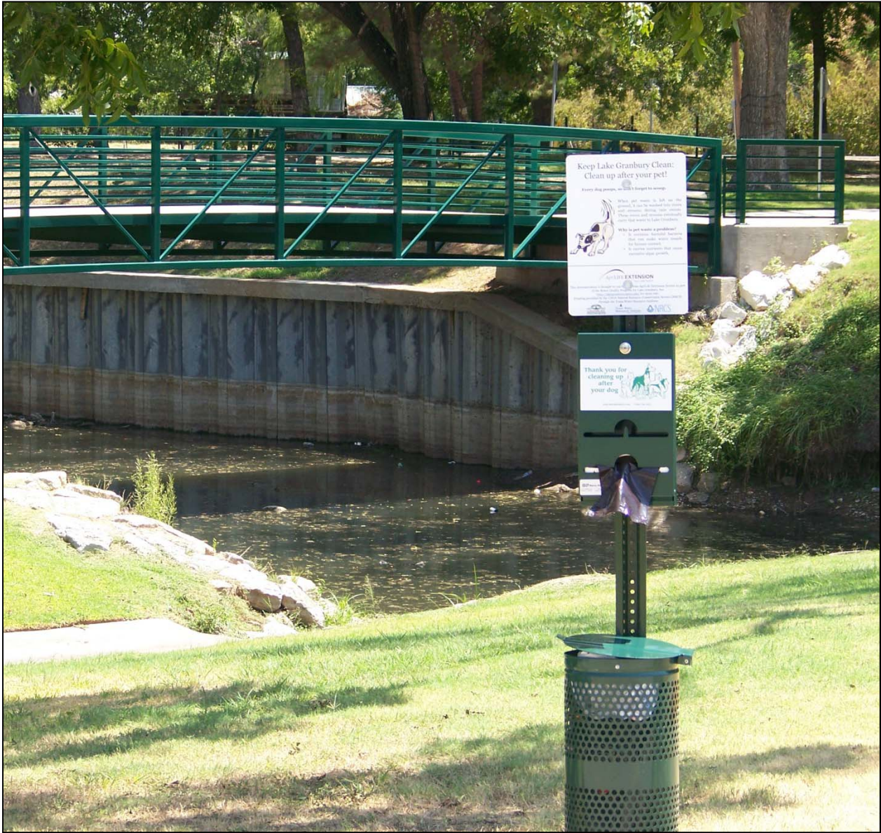
Figure B-2. Picture of the pet waste station installed along the Hike and Bike Trail near downtown Granbury.
