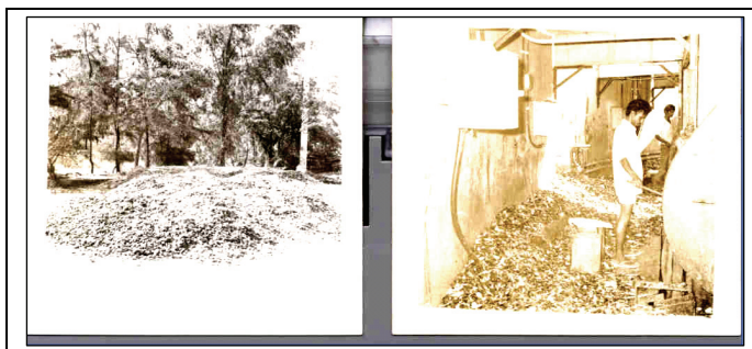
Fig. 1. Removed fouling organisms from the tunnel of a seawater cooled nuclear power plant (Madras Atomic Power Station) by shock chlorination
