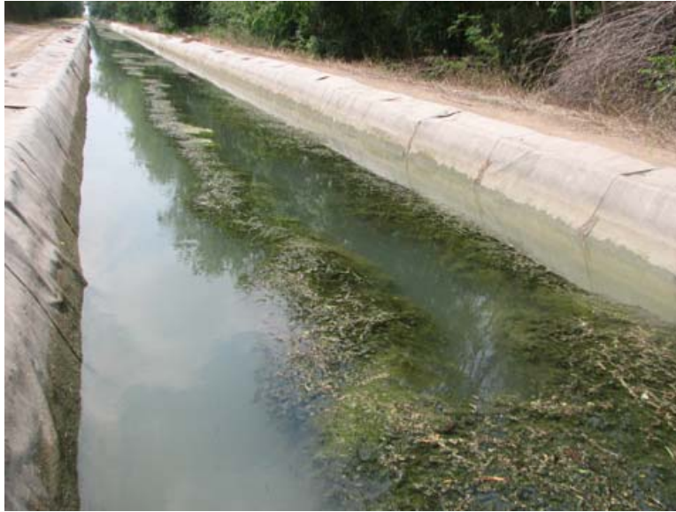
Fig. 4.10. Hydrilla verticillata growing in a channel with maintained water depth and no flow. (at time of photo)
