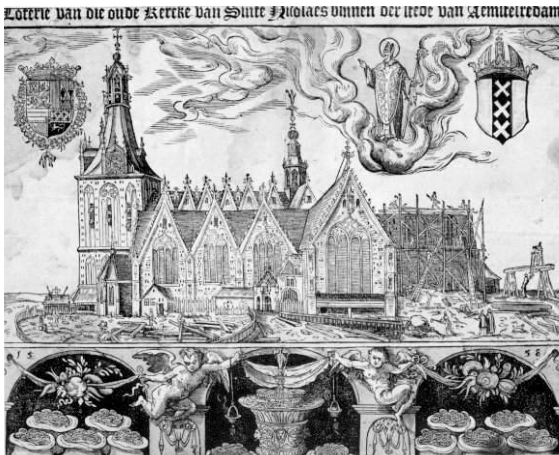
Fig. IV.91 Two sawyers working a framed pit saw. Lottery ticket, Old Church Amsterdam, 1548.
