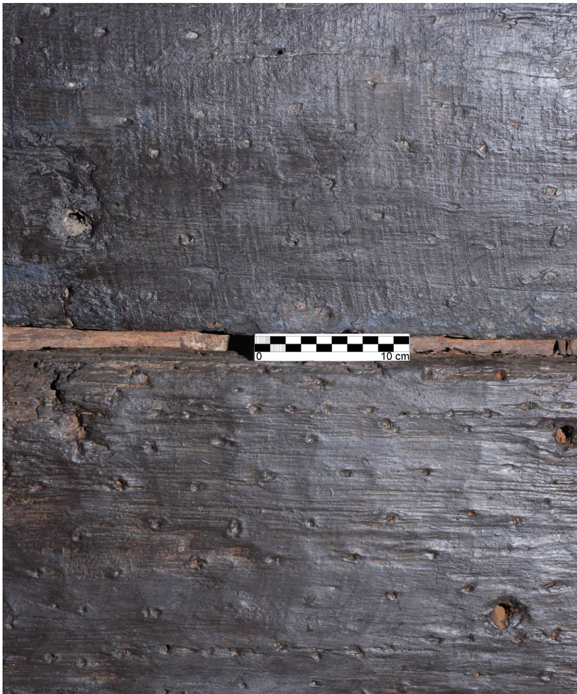
Fig. IV.93 Outer layer of hull planking with saw marks of framed pit saw (top) and adze marks (bottom), Batavia shipwreck, BAT 6078 (top), Strake 13, and BAT 6106 (bottom), Strake 12. Photograph: Patrick Baker, Western Australian Museum.
