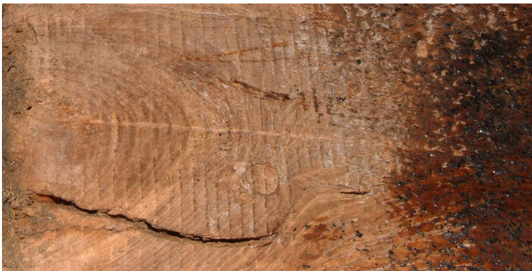
Fig. V.40 Saw marks on pine joist used in the construction of sawmill, De Rat , in IJlst, Netherlands, sawn mechanically by wind-driven sawing mill (17 saw marks per 0.010 m), dating to 1683 or earlier. Photograph: Simon Jellema, miller of De Rat .
