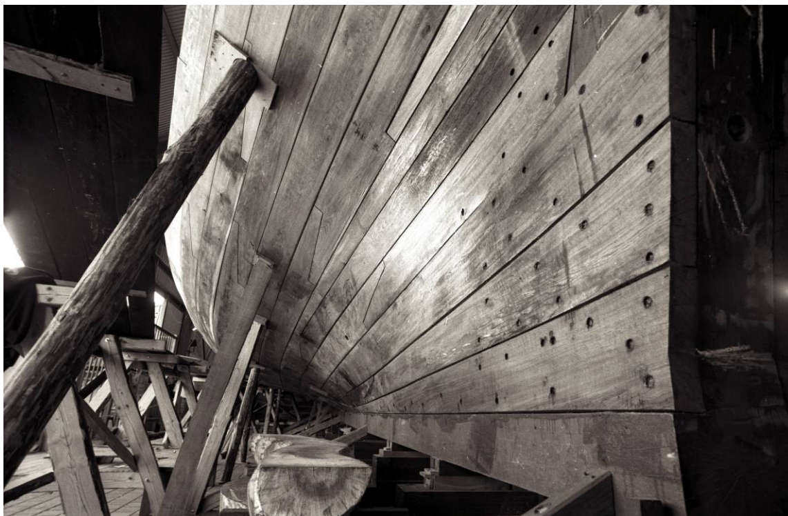
Fig. IV.27 The use of wooden shoring poles on the outside of the ship's hull to support its planking, reconstruction of VOC ship Duifje , 1606. Photograph: Patrick Baker, Western Australian Museum.
