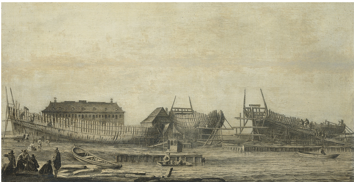
Fig. II.18 The shipyard of the Amsterdam Admiralty with three warships being constructed in a frame-first method. Ink on Painting: Ludolf Bakhuysen, 1655–60, Rijksmuseum Amsterdam (SK-A-1428).
