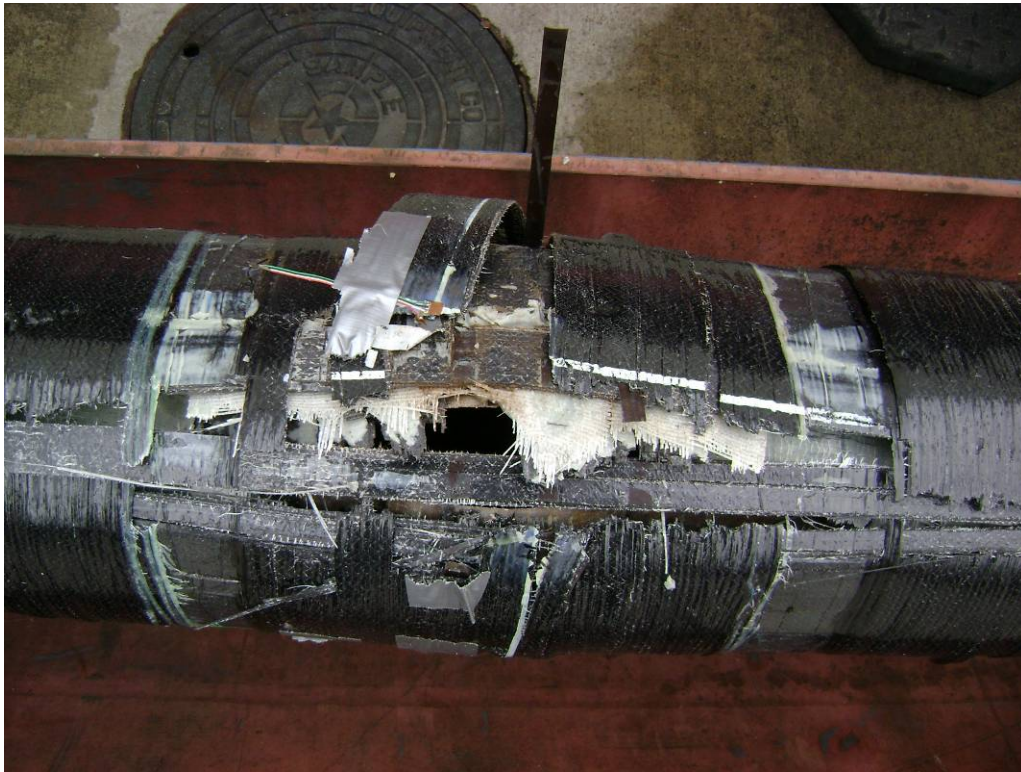
Figure 68 – Photo of burst test sample showing failure
