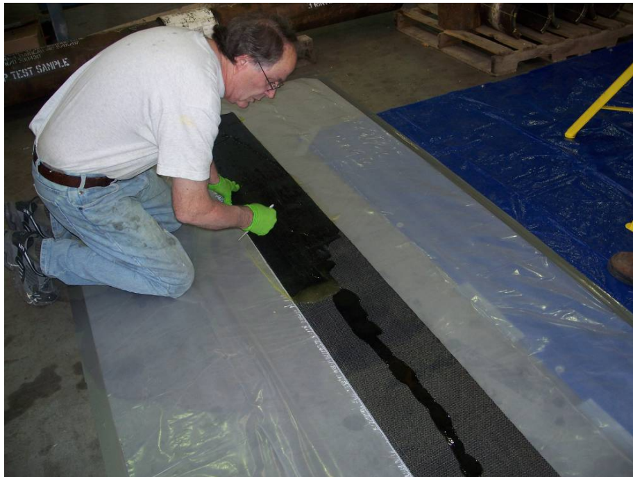
Figure 47 – Saturating the uniaxial stitched carbon cloth
