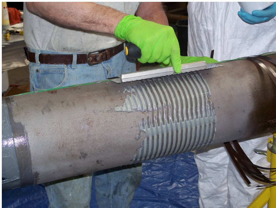
Figure 51 – Applying the epoxy adhesive using a slotted hand trowel
