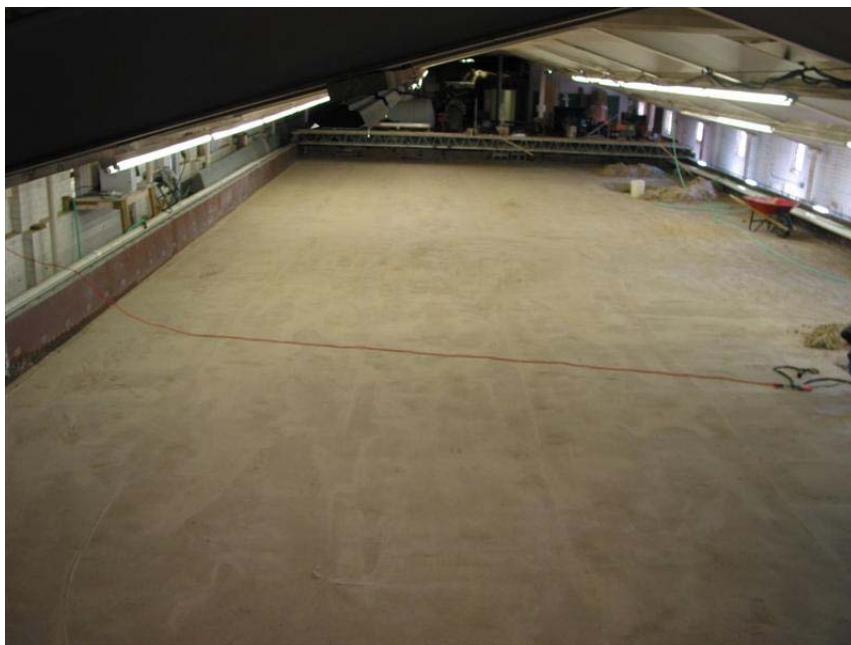
Figure A.4 Completion of Leveling Work
