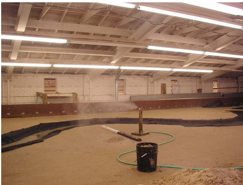
Figure A.8 Sprinkling the Clay Banks
