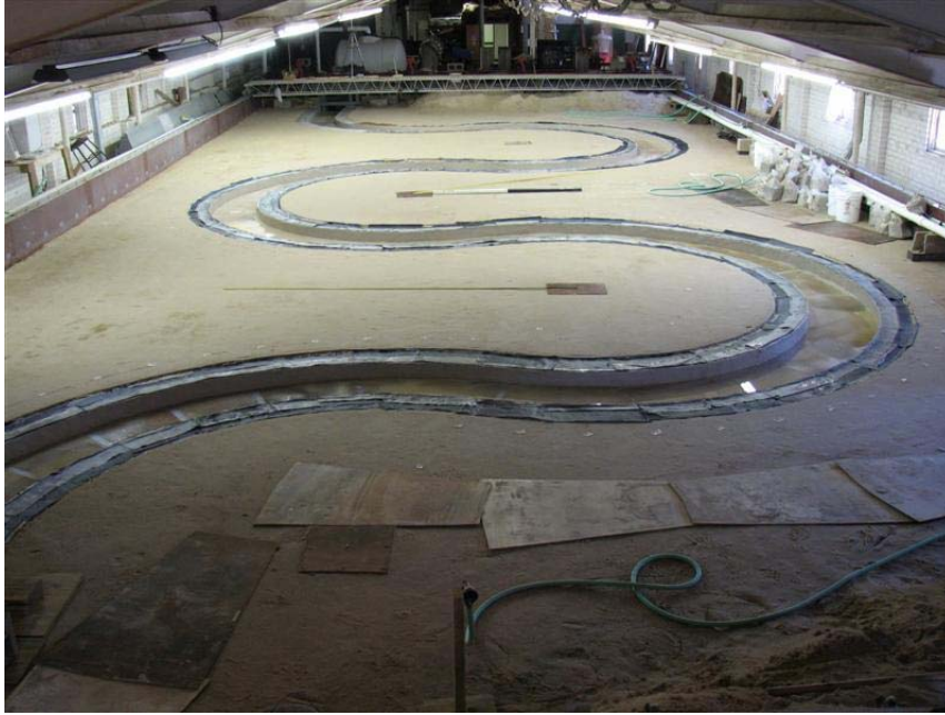
Figure A.9 Completion of the Clay Channel
