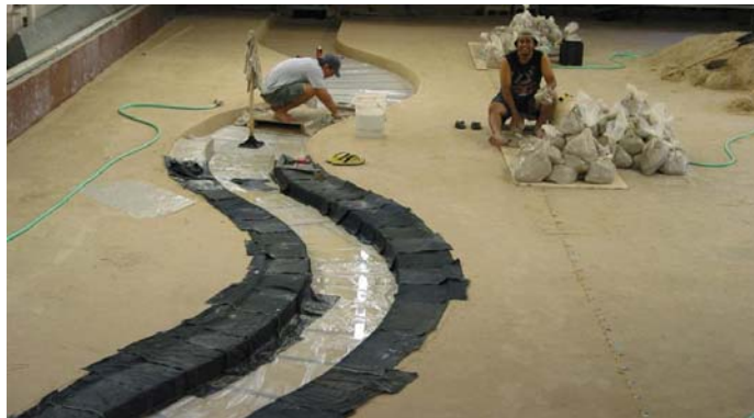
Figure 4.19 Laying the Clay Blocks along the Channel
