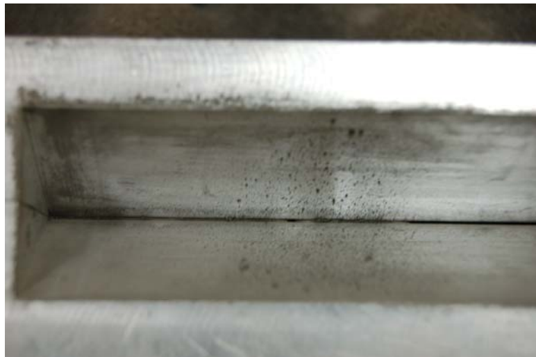
Figure 6.2. Clogging of LSVI nozzles due to heavy mass loading
