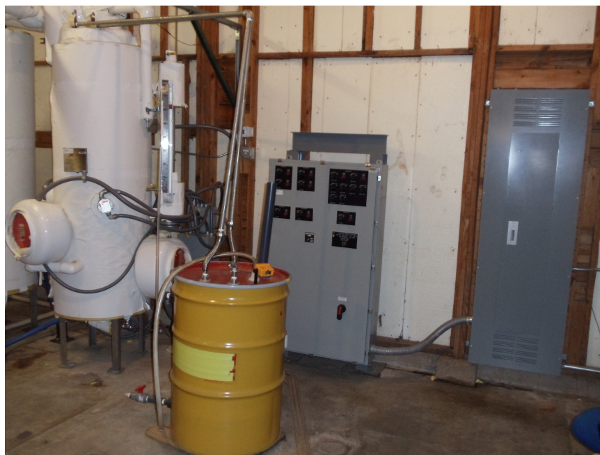
Fig. 3.3.: The steam generator and associated components.
