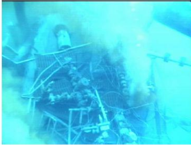
Fig. 4 –Underwater photo of a toppled platform in the Eugene Island Area (BOEMRE, 2007).
