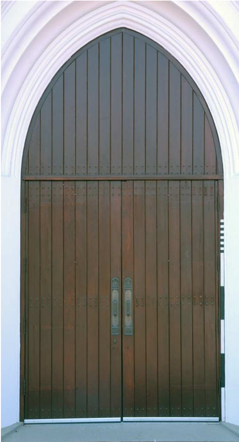
Fig. 11. A reference scale was placed next to the entryway of St. Andrews church when the CHC team documented the church in 2010. Note the scale located at the right side of the door. (Copyright: Center for Heritage Conservation.)
