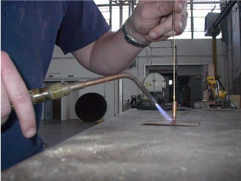
Figure 9. Soldering of copper tubing
