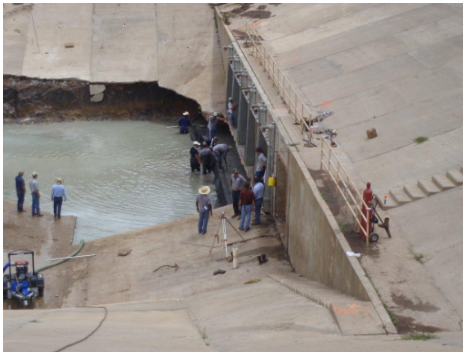
Figure 4.1. Pictures of drop structure before (a) and during (b) emergency stabilization efforts. Photos are reproduced (FNI 2011a) with permission of FNI and client.
