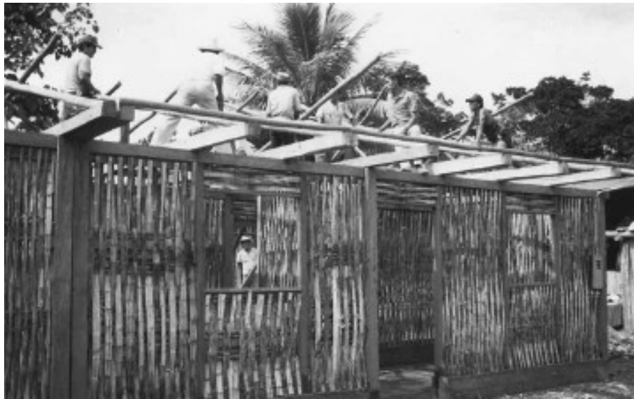
Figure 23. Quincha house under construction in Alto Mayo, Peru. Source: Schilderman, 1993.
