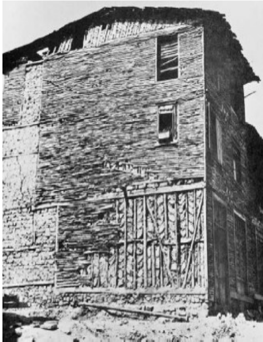
Figure 22. Timber framed ground floor of an undamaged building in Akcaalan, Turkey. Source: Gülhan, 2007.
