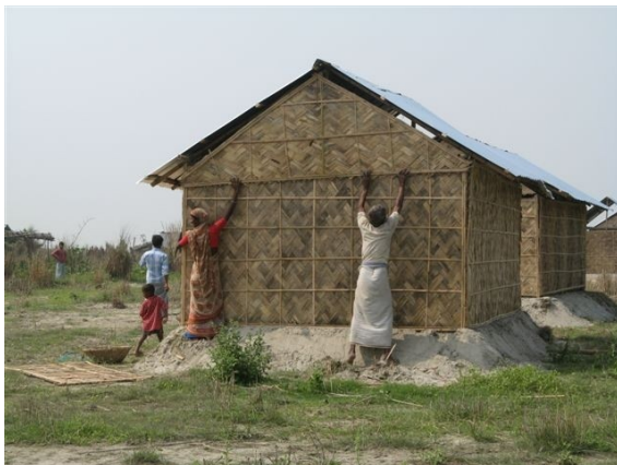
Figure 25. Raised platform flood prone house in Bangladesh. Source: Hufstader, 2008.
