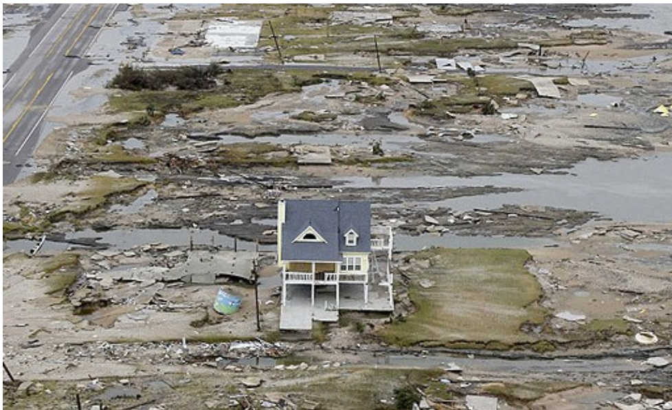
Figure 29. The structure called “Last House Standing” in Gilchrist was built by the owners after Hurricane Rita. Source: IBHS, 2009.
