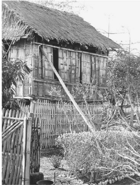
Figure 24. Use of bamboo poles to brace structures during storms in Philippines. Source: Schilderman, 2004.
