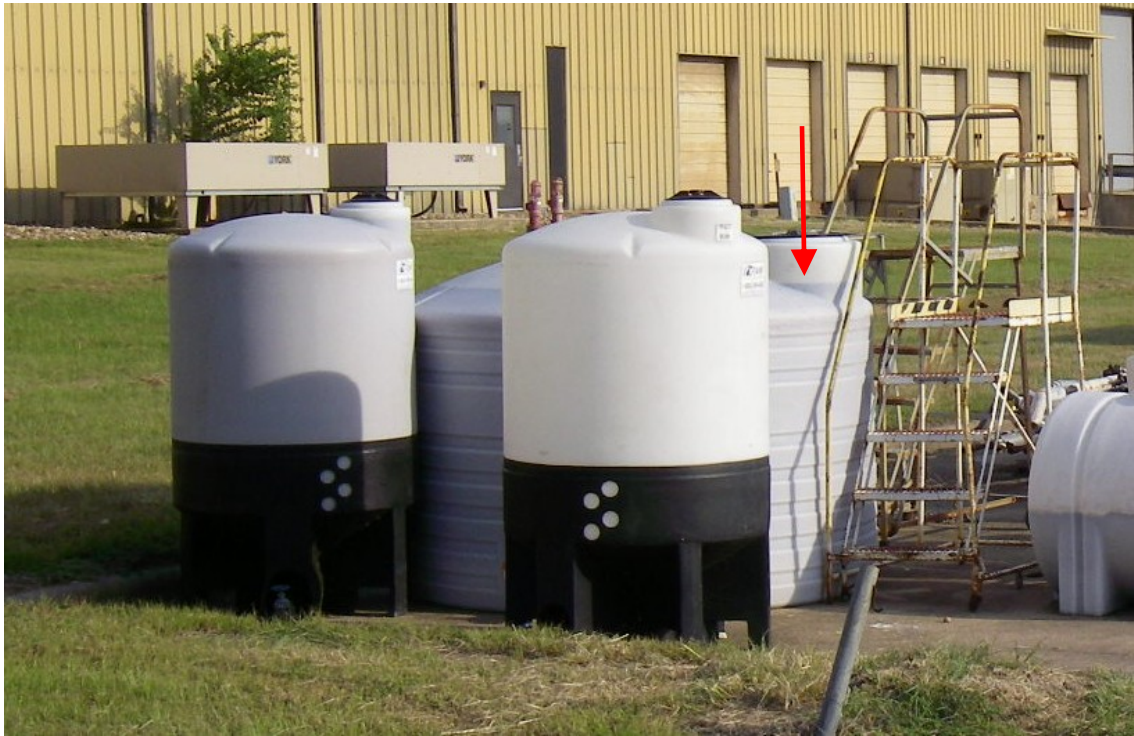
Figure 2-29. Plastic tanks used to storage fermentation product liquor. The red arrow indicates the storage tank with the product liquor that was monitor.
