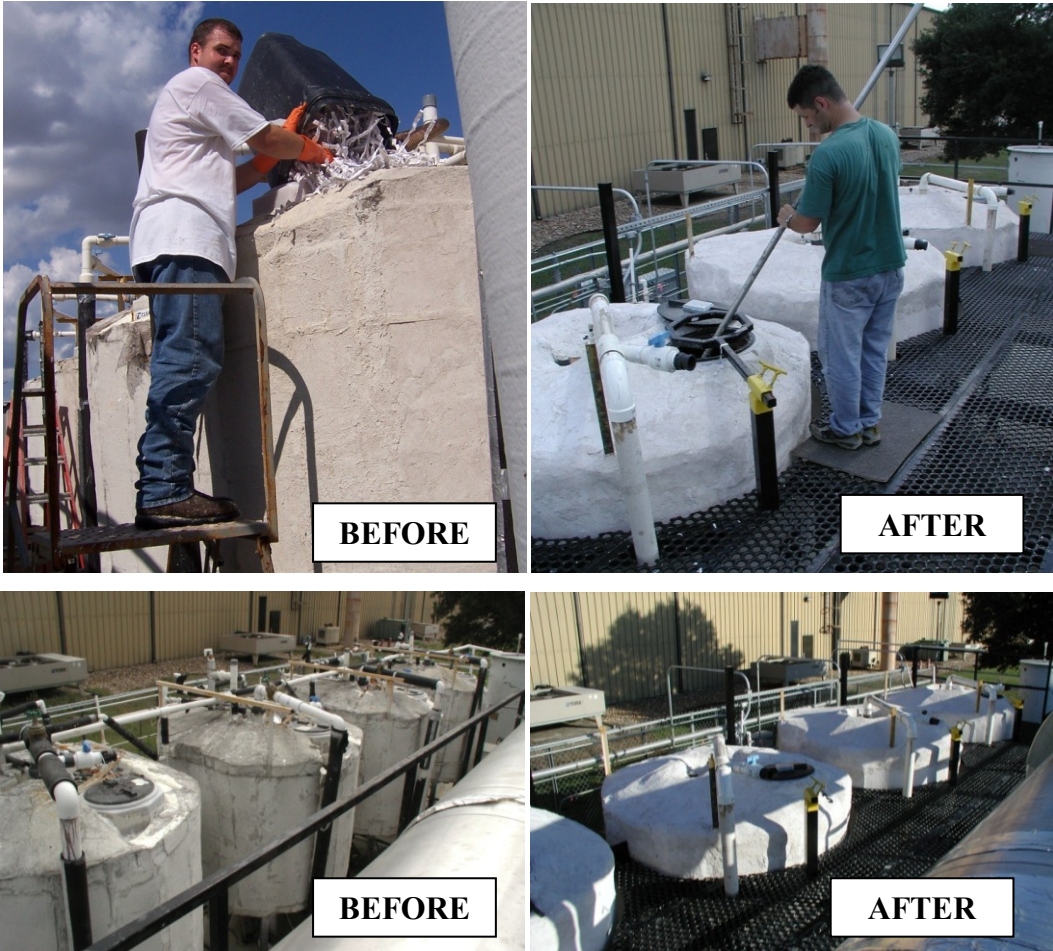
Figure 2-8. Pictures of fermentor access before and after catwalk construction.
