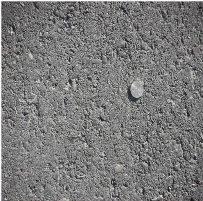
FIGURE 150 Type C mixture on shoulder of SH 16 in San Antonio District.
