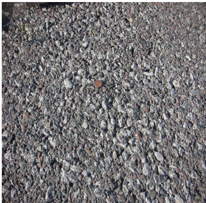
FIGURE 145 CMHB mixture on wheelpath of US 87 in Lubbock District.
