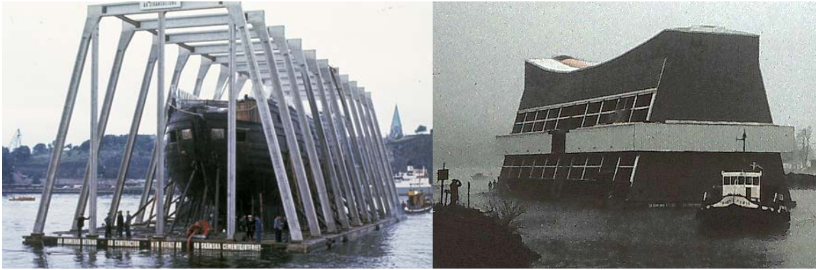
Figure 5. Superstructure built over the Vasa on the floating pontoon. Left, superstructure of concrete beams; Right, final enclosed superstructure (Courtesy Archives, the Swedish National Maritime Museums).
