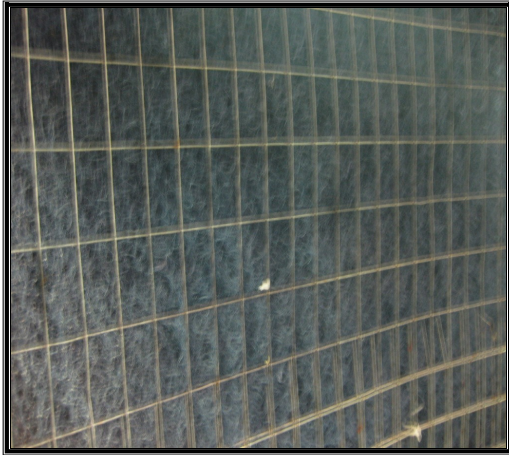
Figure 18. Net used to prevent fine sand from leaving the tank when water is drained to reform sand bed after bed leveling.
