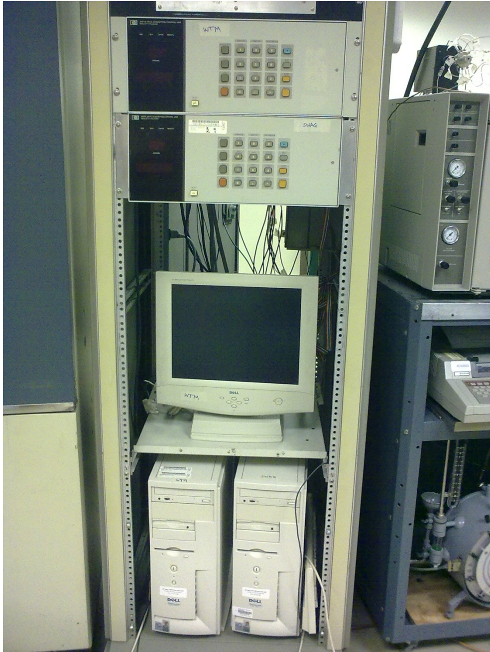
Fig. 3.12 – Data logger unit and PC.
