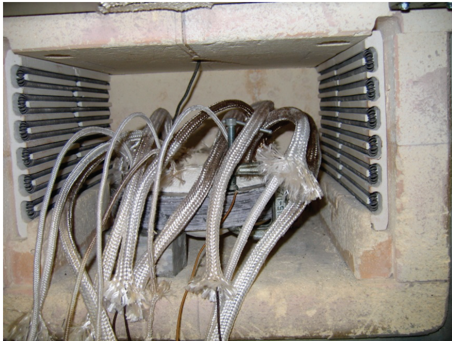
Fig. 4-1 Motor Stator in Oven for High Potential Test
