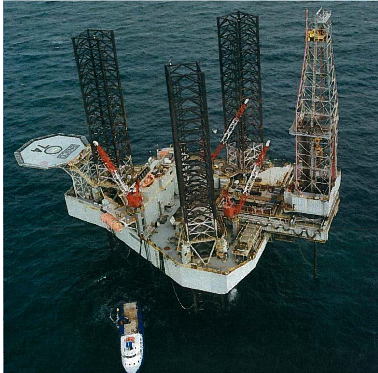
Figure 1.1 Mobile jack-up unit (courtesy of LeTourneau Inc.)
