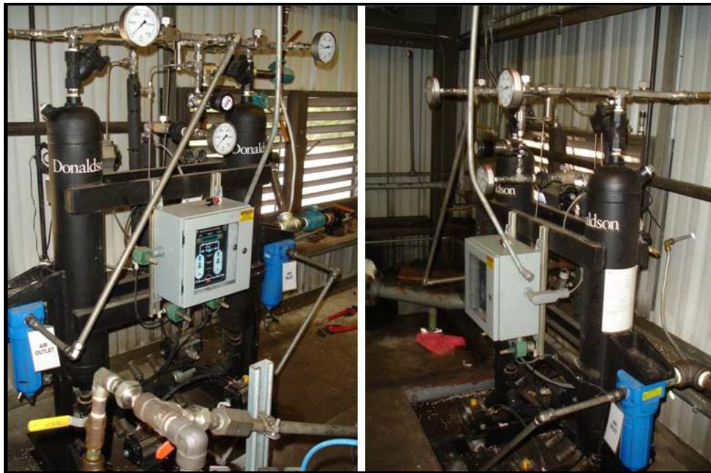
Figure 12: Donaldson High Pressure Air Dryer
