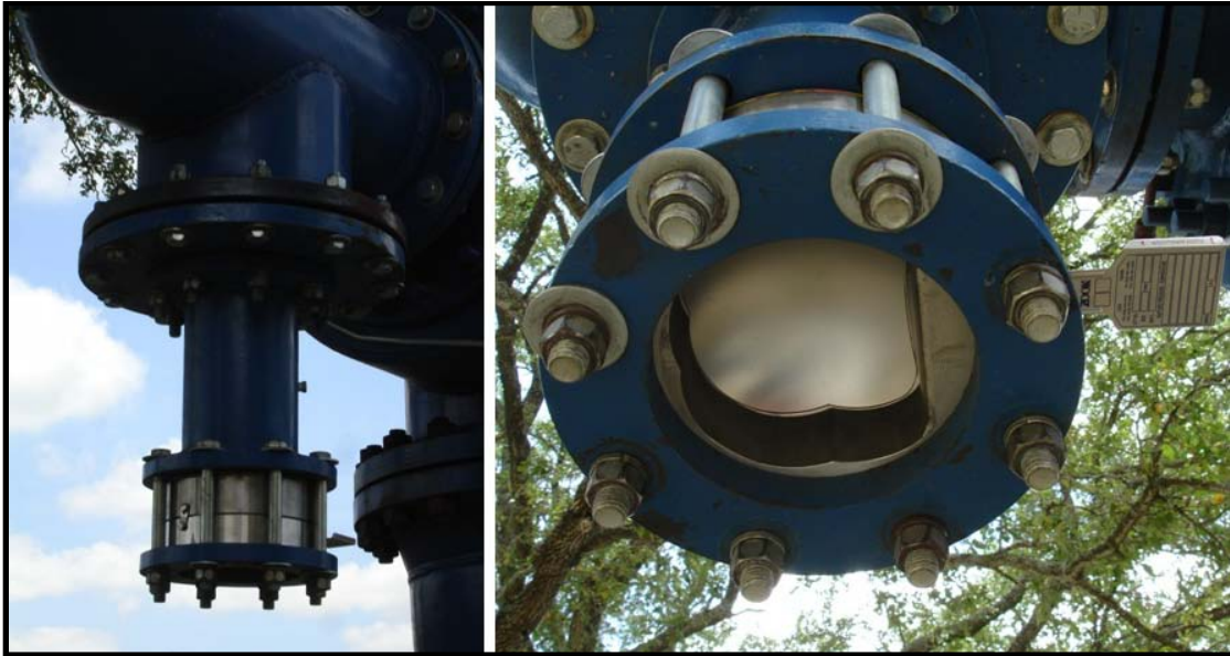
Figure F-10: Second Stage Rupture Disk System
