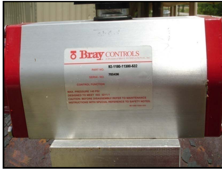
Figure 27: 2" Tank Actuator
