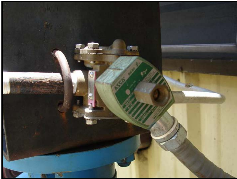
Figure 21: ASCO 3-Way Solenoid Valve
