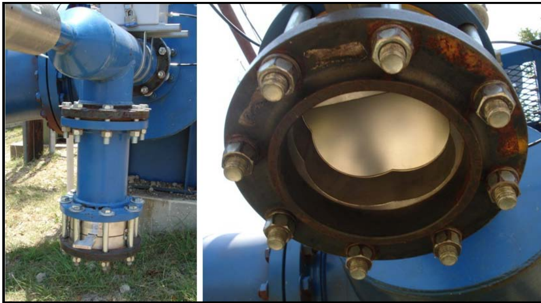
Figure F-9: First Stage Rupture Disk System
