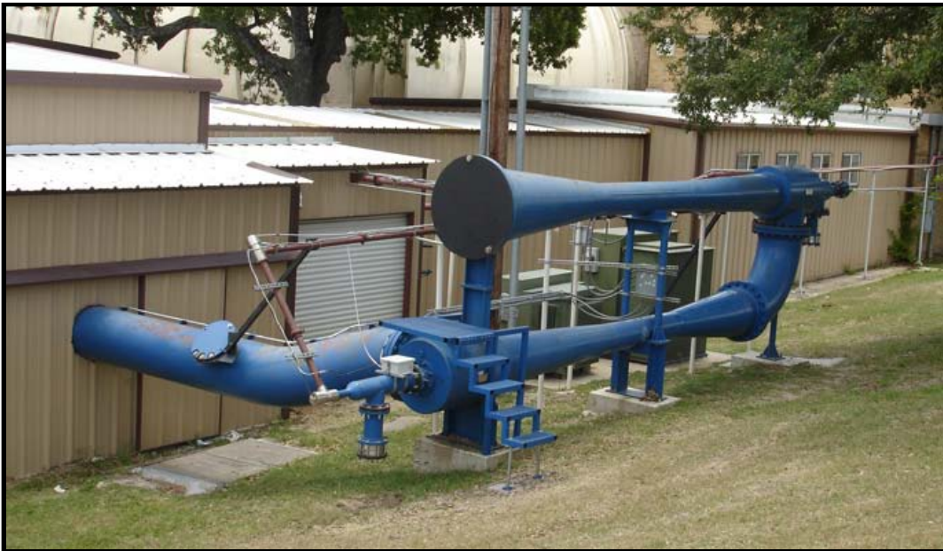
Figure F-21: Fox 2-Stage Air Ejector
