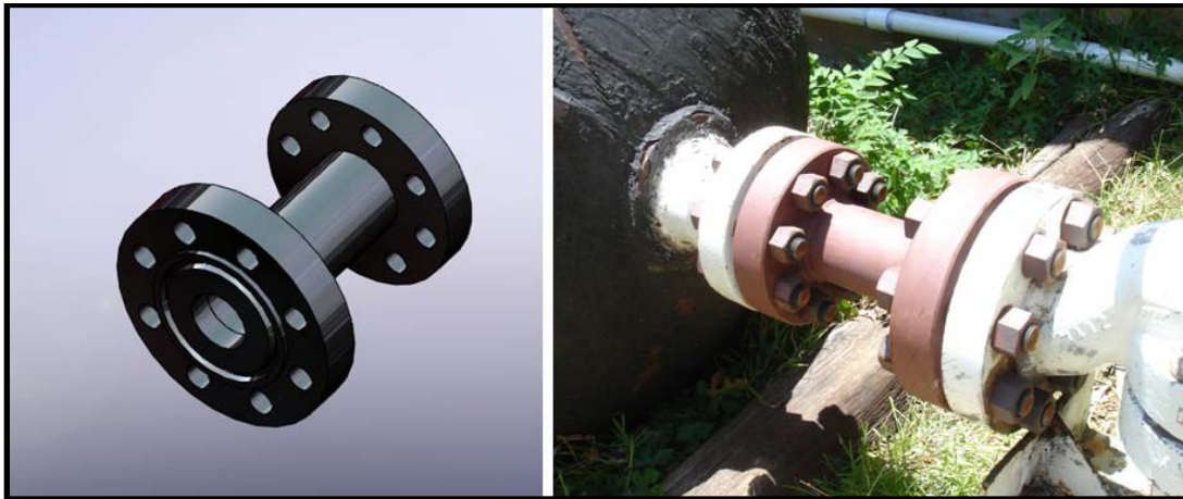
Figure 15: New Tank Exit Contraction Section
