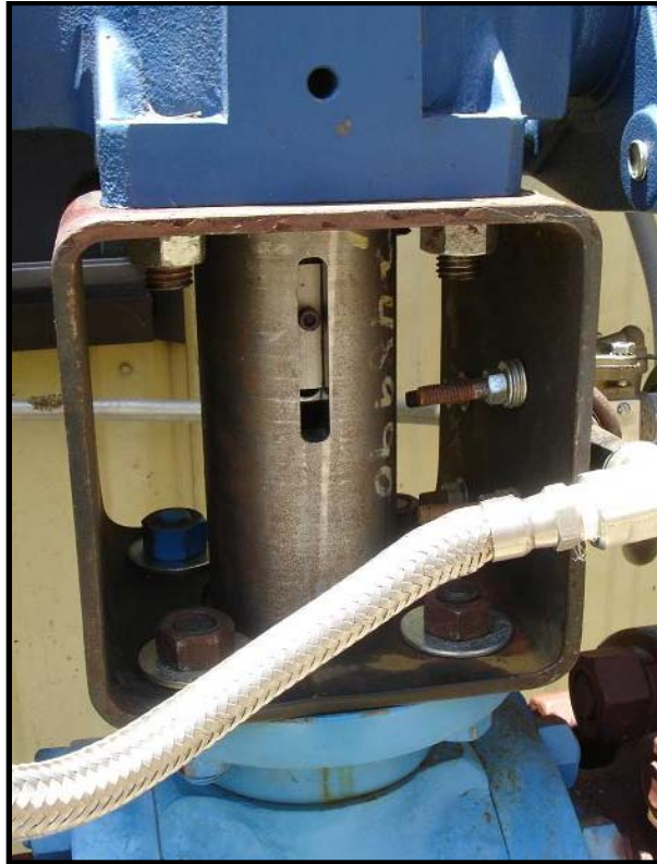
Figure 20: 4" Actuator Mounting Shaft
