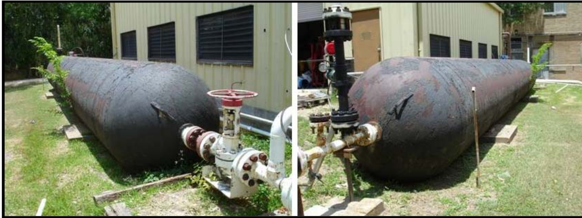
Figure 14: A. D. Smith High Pressure Storage Tank
