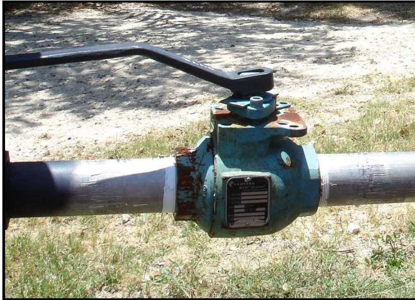
Figure 26: 2" High Pressure Ball Valve
