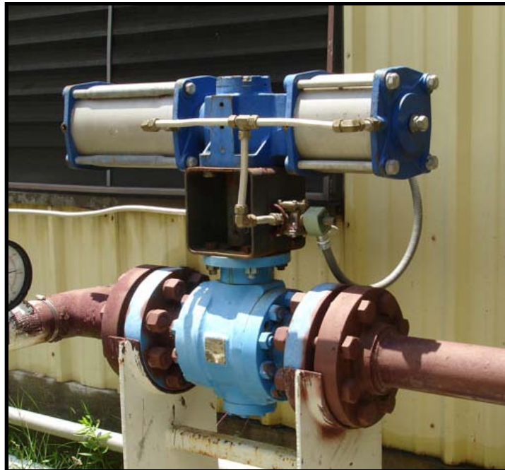
Figure 17: Original Actuator and Ball Valve
