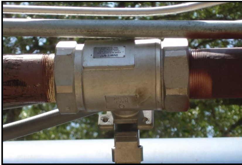
Figure F-3: First Stage Ball valve
