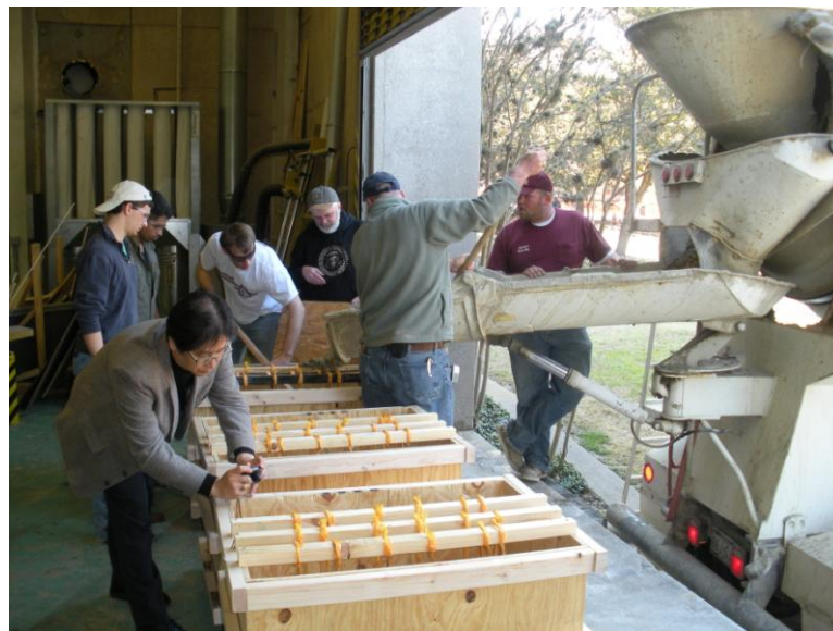
FIG. 5.5. Formwork and pouring of tags
