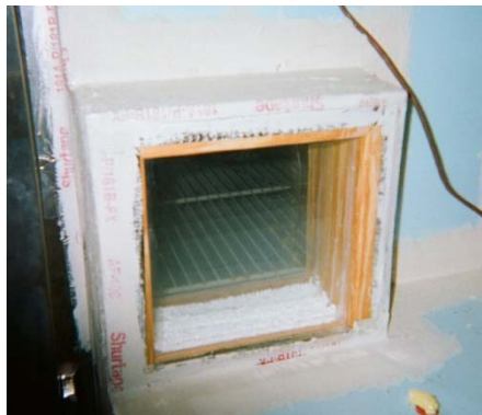
FIG. A-11. Quadruple Glazed Viewing Window
