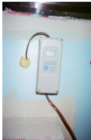
FIG. A-1. 24 Volt Commercial Thermostat Control
