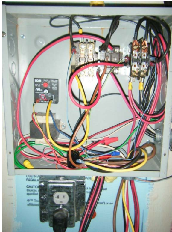
FIG. A-2. 24 Volt Electronic Temperature Control System
