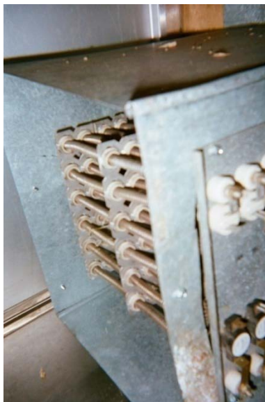
FIG. A-6. 5-Kilowatt Heating Strip Assembly
