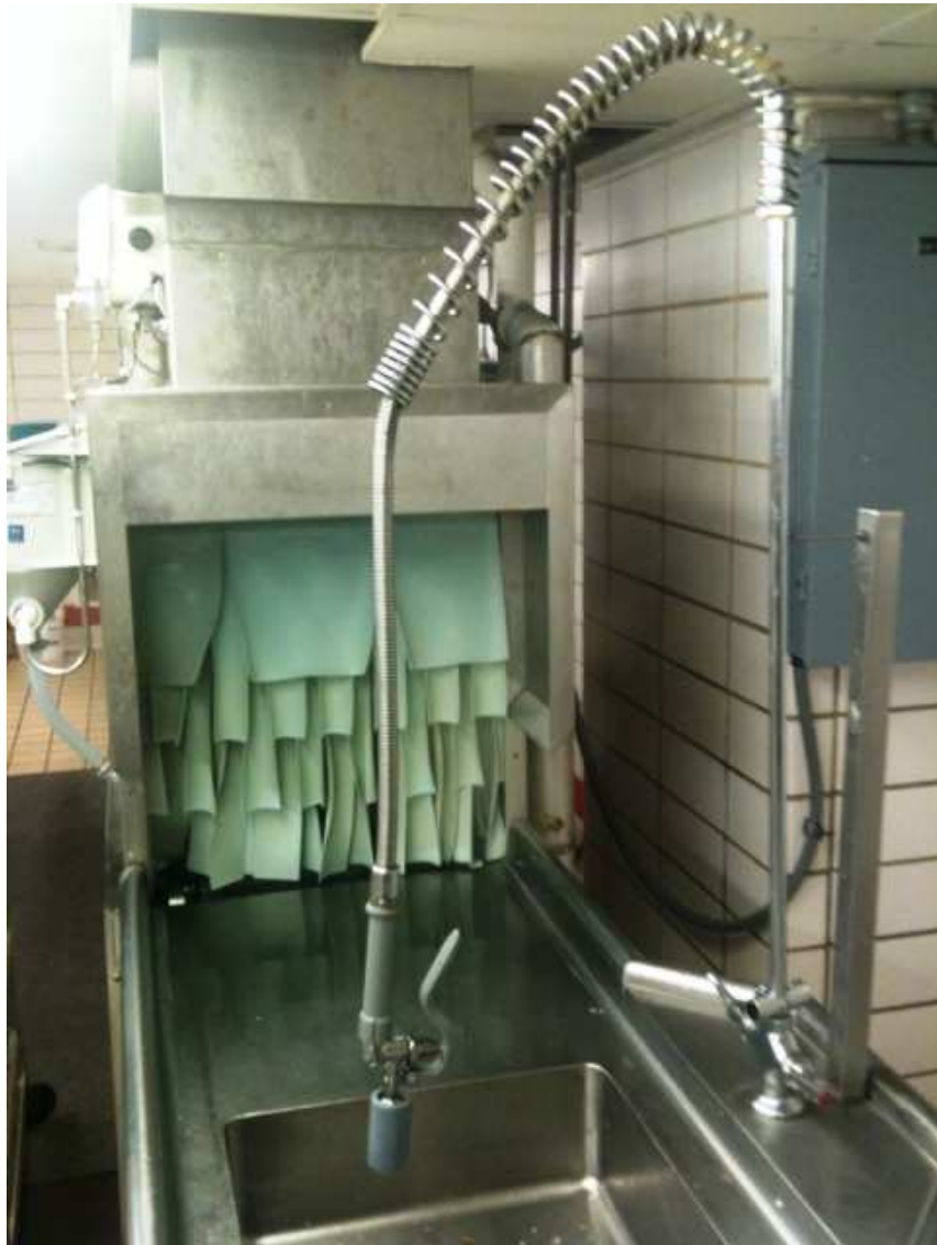
Figure2: Proposed PRSV: T & S Brass B 0107-C, 0.65 gpm at 60psi
