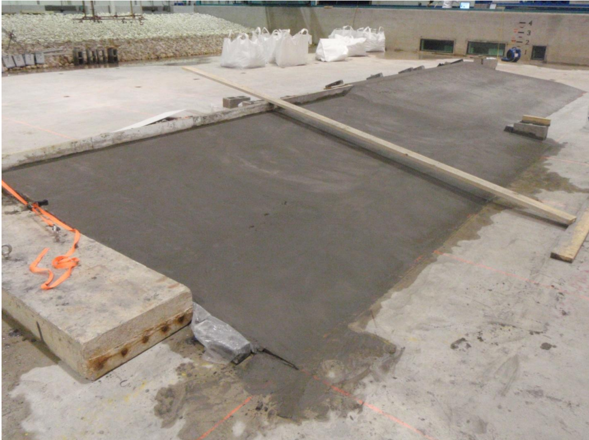
Figure 22. Finished Transition of Levee Transition Model.
