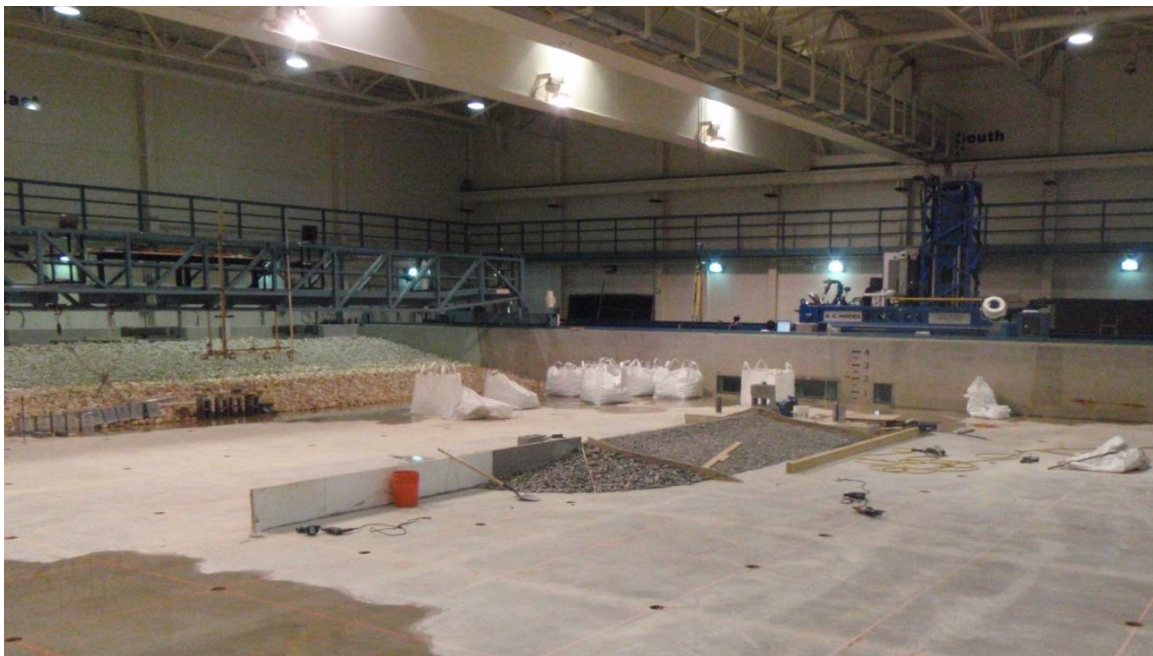
Figure 18. Initial Construction of Levee Transition Model.
