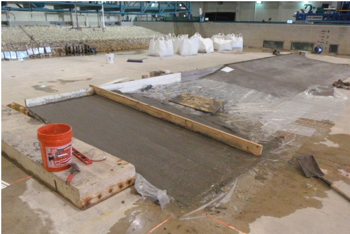
Figure 21. Placement of Concrete in Floodwall Section of Levee Transition Model.
