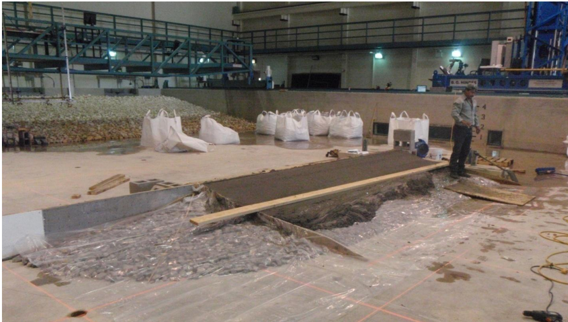
Figure 19. Placement of Concrete in Levee Transition Model.
