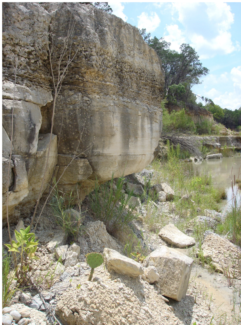
Figure 12. Photograph of rock erosion accumulation.
