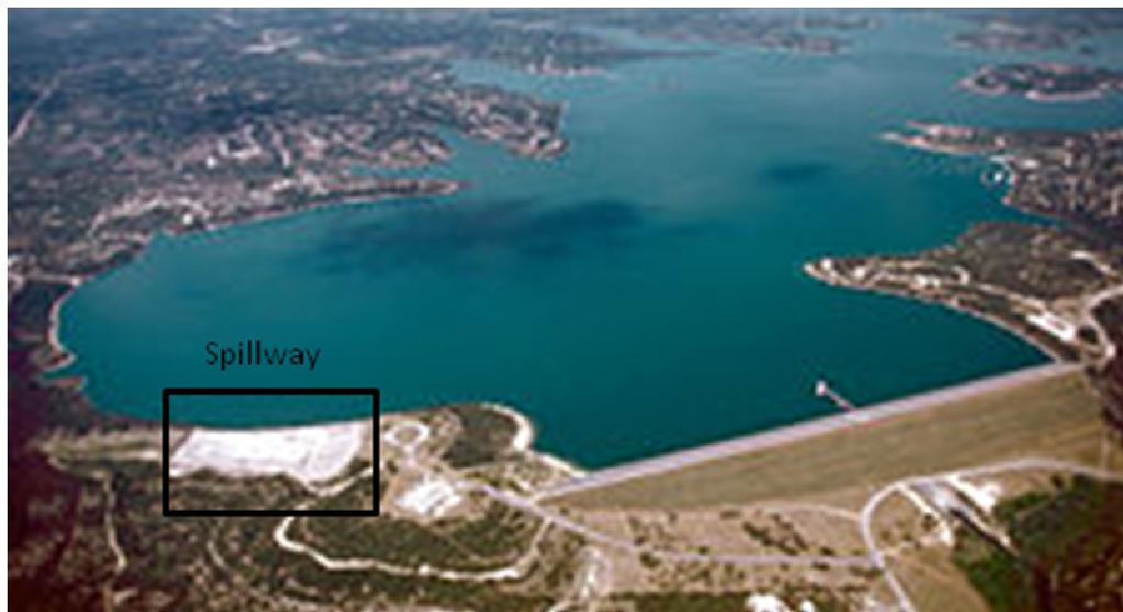
Figure 3. Pre-flood aerial photo of Canyon Lake (CCEO, 2002b). Spillway featured at bottom left, dam featured on the right. View is towards the northwest. Photo courtesy Comal County Corp of Engineers Office.
