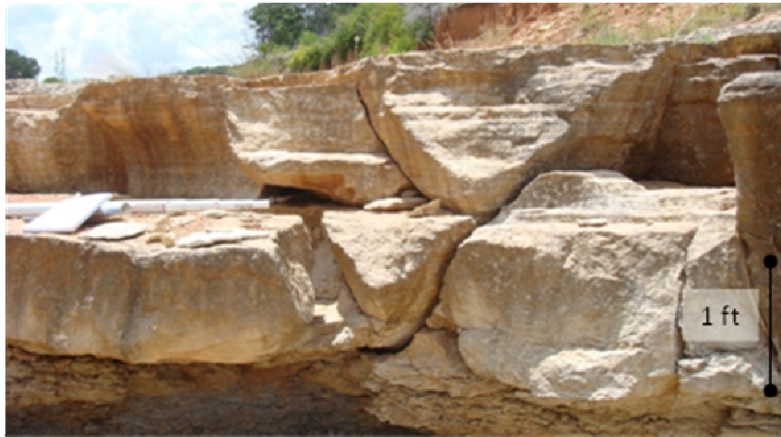
Figure 27. Rock unit 2-2. Unit 2-2 is a packstone that is 0.91 m (3.0 ft) thick. The impact test hammer averaged a rebound value of 38.43 ( 367.7 \text{ Kg/cm}^2 , 5230 psi) in seven successful measurements.
