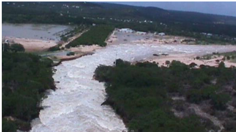
Figure 6. Photo showing flow directed over the breached spillway ( http://www.cceo.org/FloodPics/index.htm , 2002). Flow is through the shallow valley towards the Guadalupe River. View is towards the East. Comal County Engineers Office.
