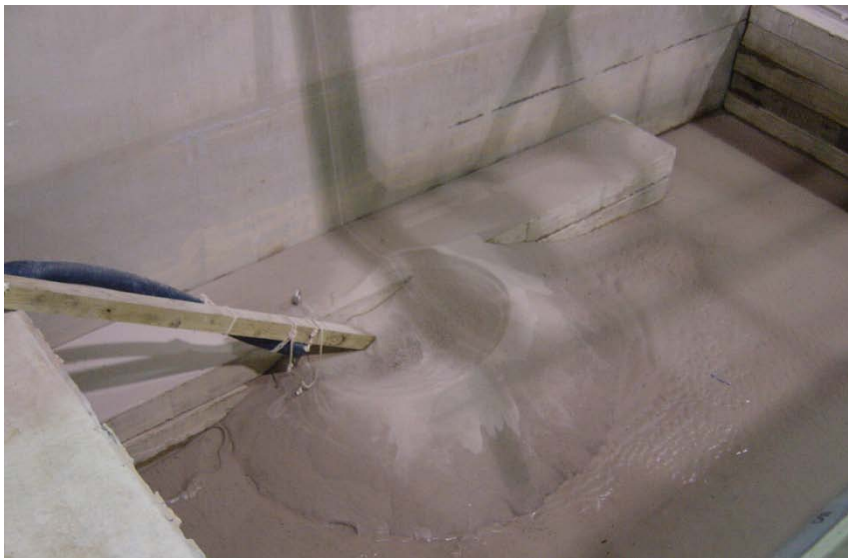
Figure 26. Confined Placement Area Post-Dredging
