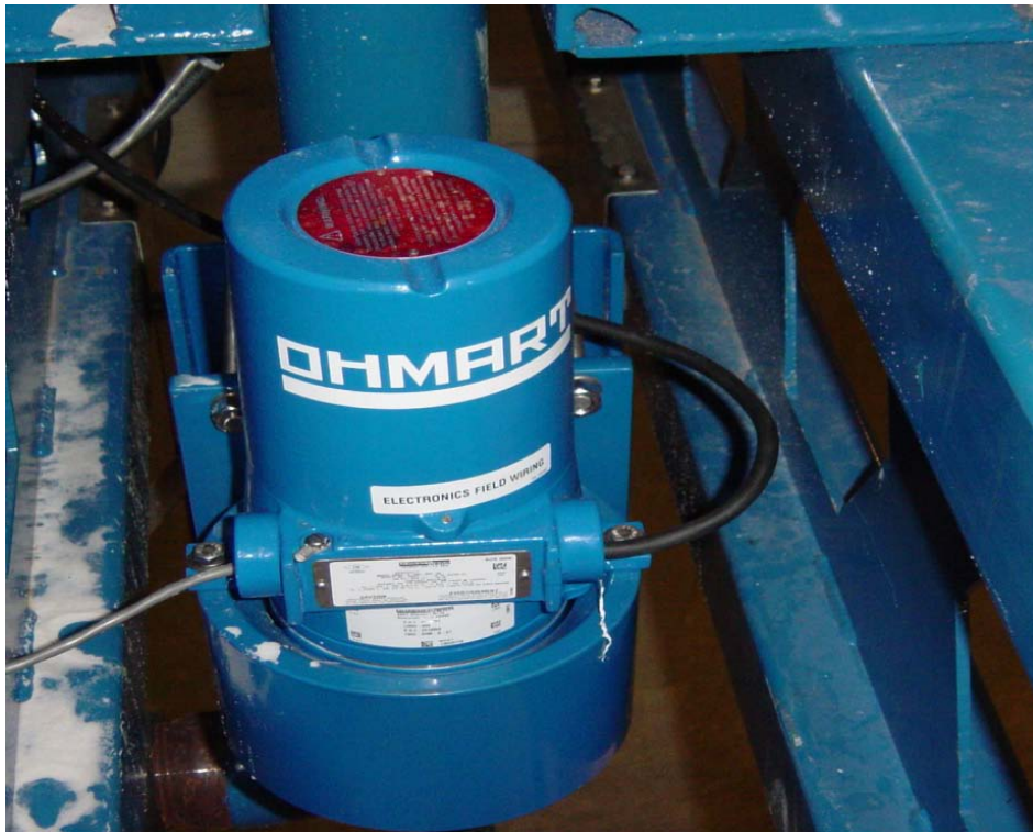
Figure 19. Ohmart Vega DSG Nuclear Density Gauge
