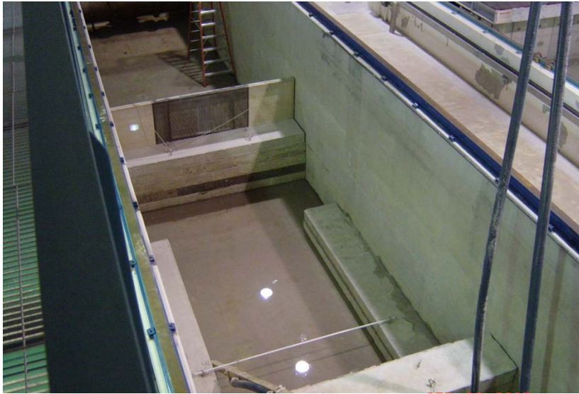
Figure 25. Confined Placement Area Pre-Dredging
