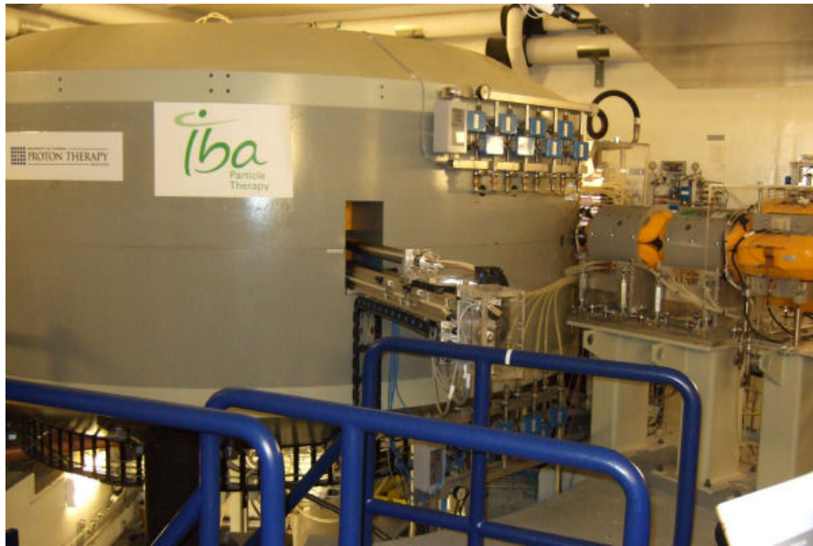
Figure 2-7. An IBA isochronous cyclotron (Medical Physics Web 2009)
