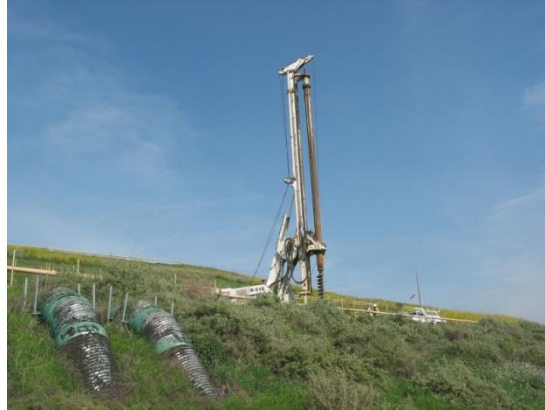
Figure 12: Drilling of LFG Collection Wells in Landfill (New Cure 2007a )
