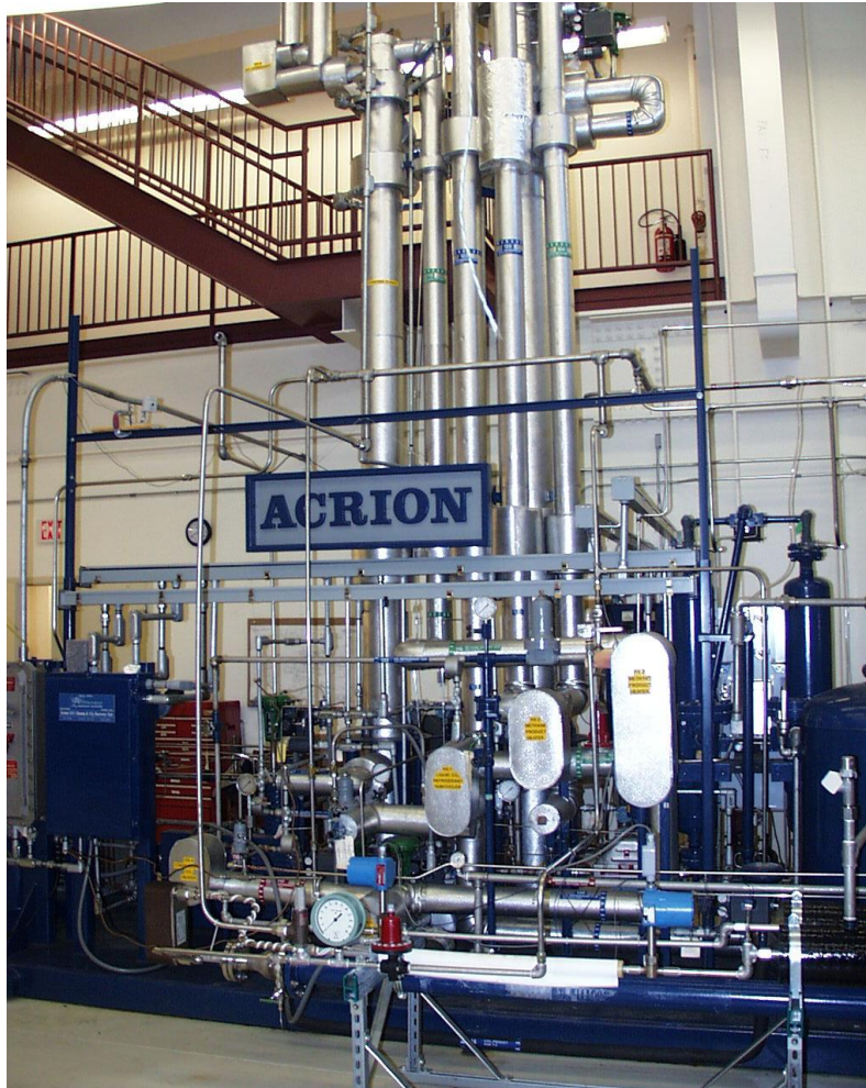
Figure 21: Acrion System at Burlington, New Jersey, Testing Facility (Cook et. al 2005)
