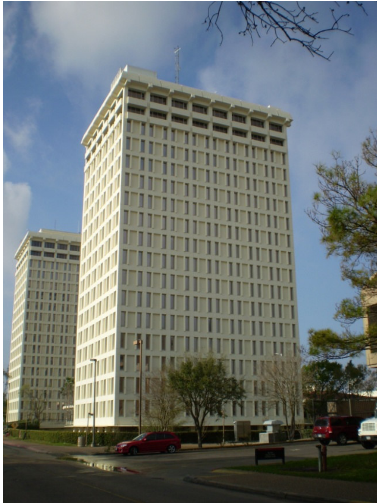
Figure 5.4. Moody Tower at the University of Houston – site for rooftop field measurements April 15 – May 31, 2009.
