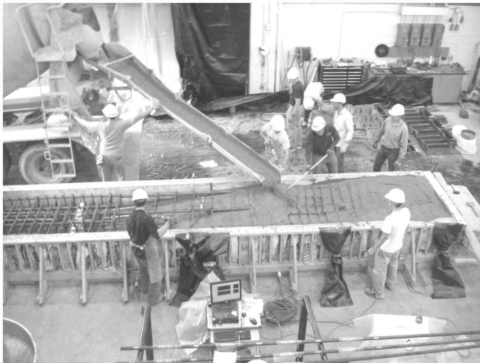
Figure 2-26 Pouring Concrete in the Form
