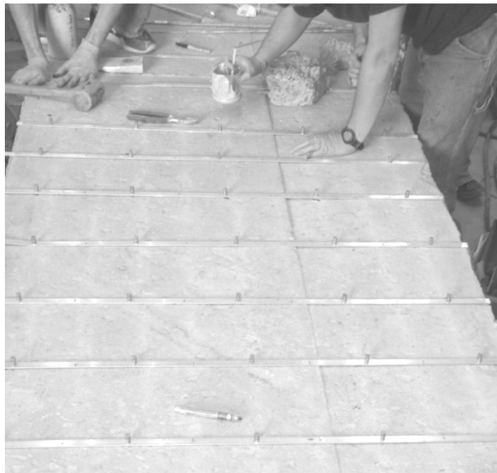
Figure 2-11 DEMEC Installation on the Long Side
