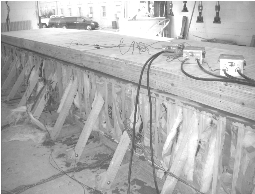
Figure 2-27 Insulated Form with ERW Power Supplies on Top
