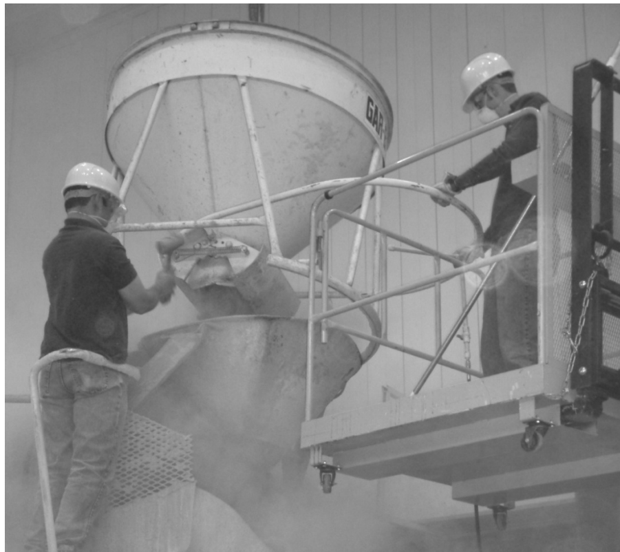
Figure 2-24 Dumping Cement into the Mixer
