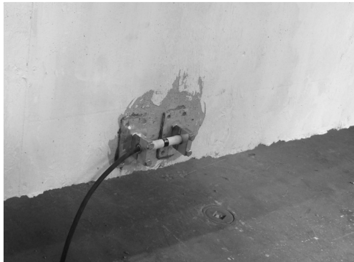
Figure 5-5 KM Gage Installation Prior to Testing
