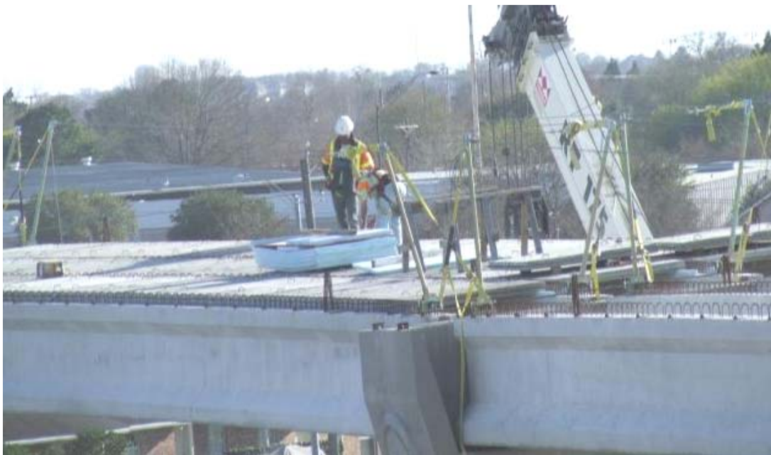
b) Placement of extruded foam and SIP panels: Jan 22- Mar 1, 2009
