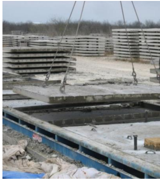
b) Lifting SIP panels out of steel forms
