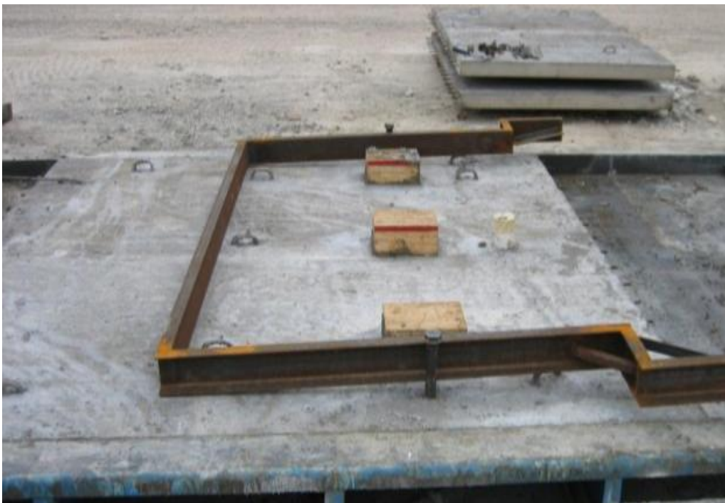
b) Steel forms for Stage II reinforced concrete pour
