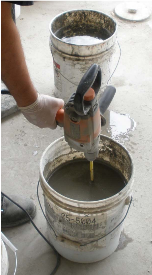
(a) Mixing of grout
