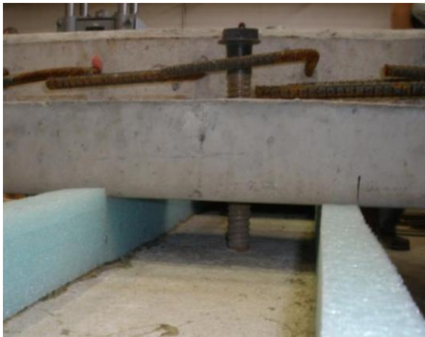
Fig. 14. Leveling bolt and haunch forming for full-depth precast overhang
