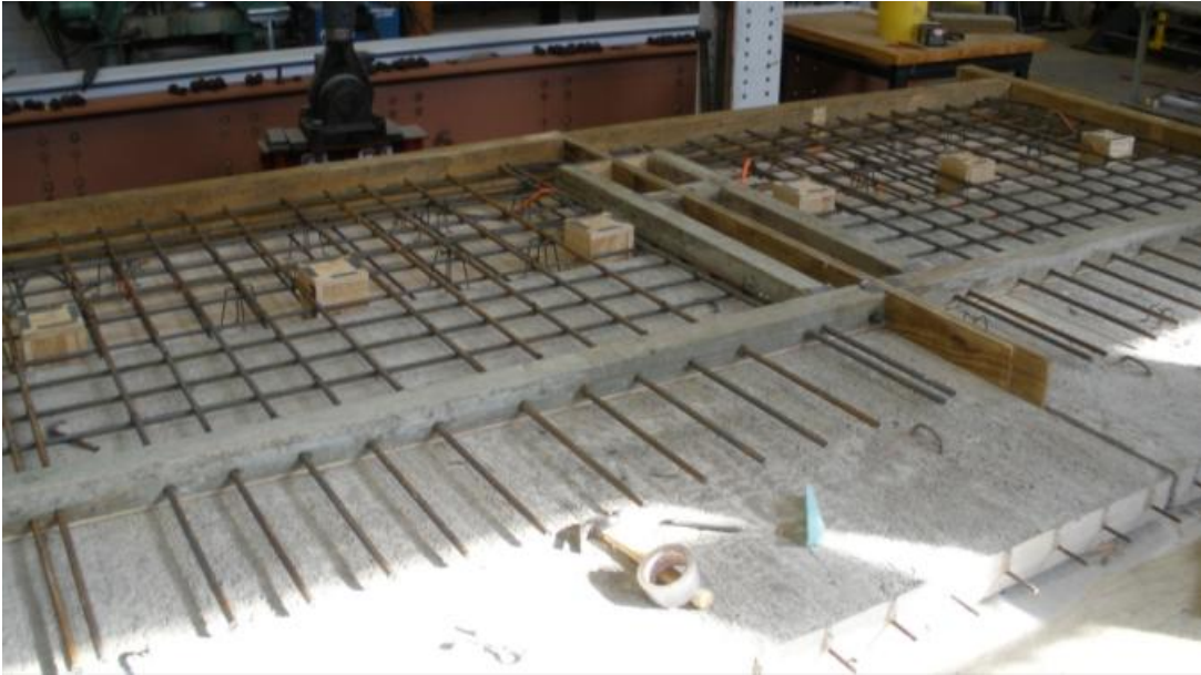
c) Transverse bars extending beyond notched forms for lap splices
