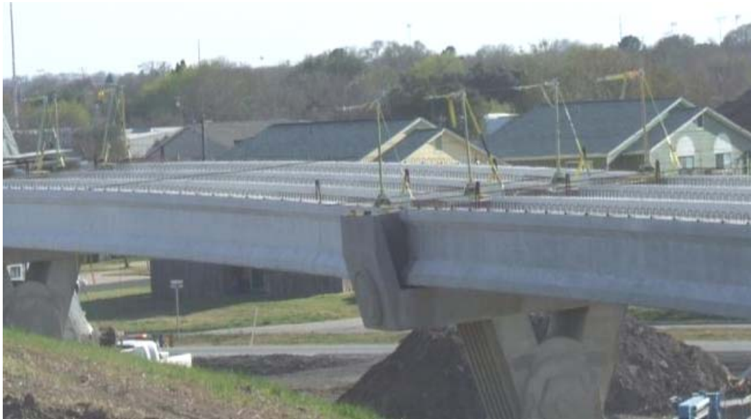
a) Placement of precast prestressed concrete girders: Jan 15-Jan 22, 2009
