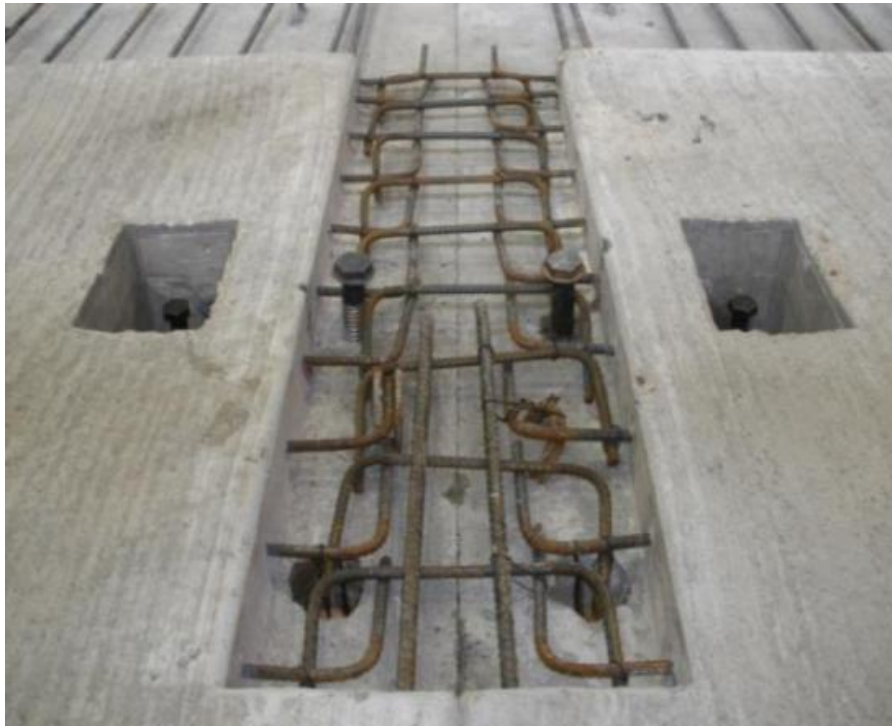
Fig. 12. Full-depth overhang panel-to-panel seam
