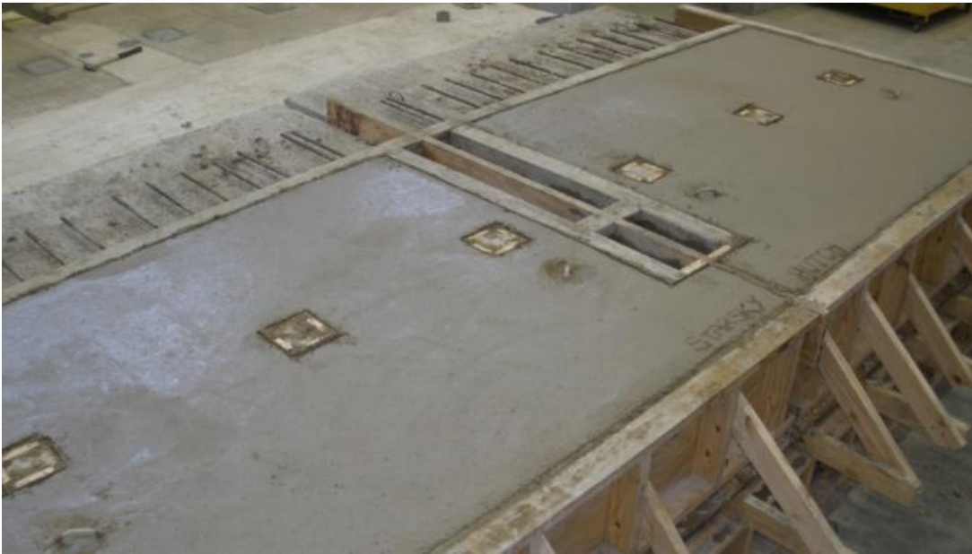
d) Completed lab-cast panels following concrete pour
