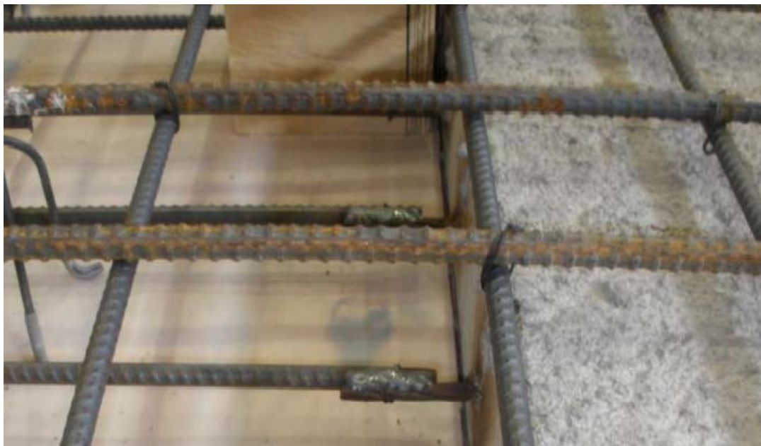
b) Bottom transverse steel welded to strand extensions
