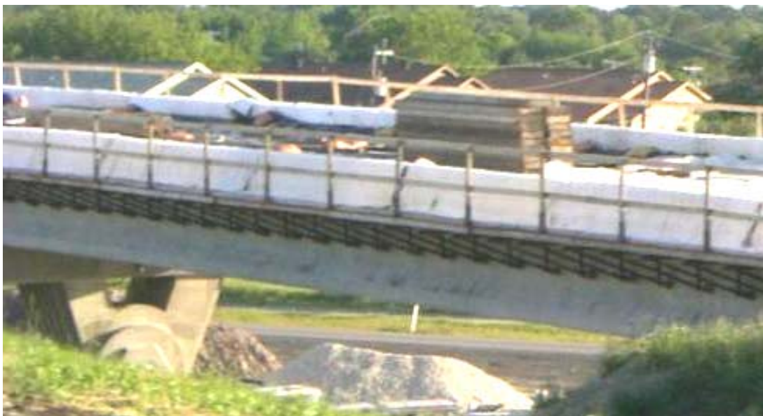
d) One day after final bridge deck pour: Apr 10, 2009
