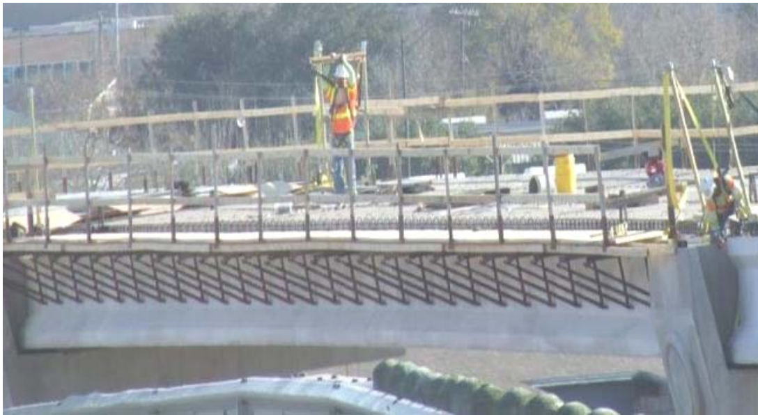
c) Overhang formwork attached (without deck walls): Feb 1-Mar 20, 2009
