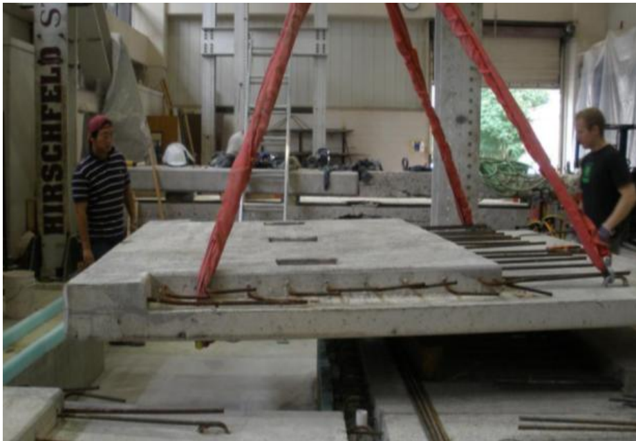
d) Placement of full-depth overhang panel on concrete girders
