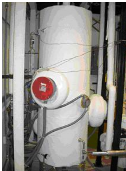
Fig. 4.6.: The steam generator after insulation.
