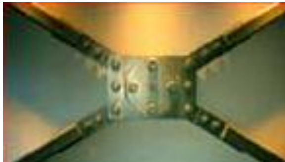
Figure 2.9: X-braced friction damper (PDL)
