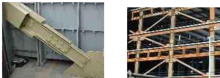
Figure 2.10: Diagonal tension/compression braced friction damper (PDL)
