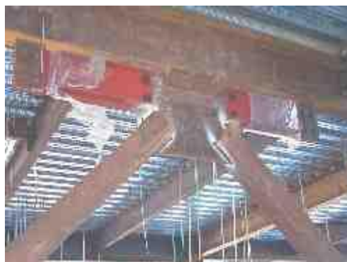
Figure 2.11: Chevron-braced friction damper (PDL)
