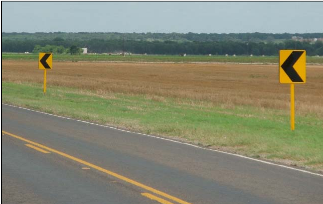
Figure 8 ChevFull Treatment on Site 2
