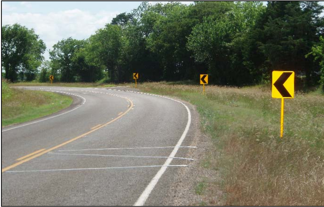
Figure 7 ChevFull Treatment on Site 1
