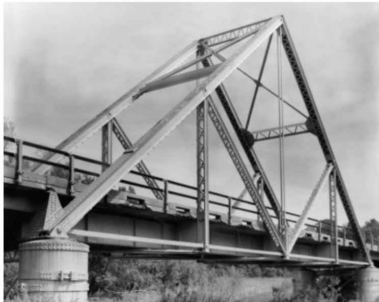
Figure 1.1 Configuration of Waddell "A" Truss Bridge.
