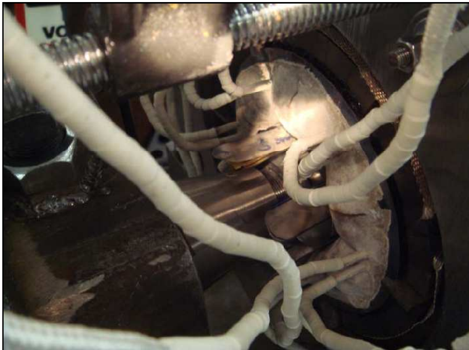
Figure 3-17 Metal shims between shaft and stator
