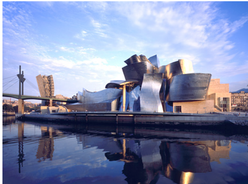
Figure 2.2 Guggenheim Museum Bilbao, Spain
