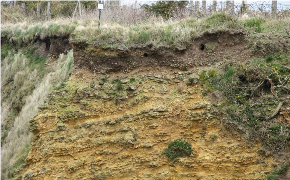
Figure 2.7. Exposed by a recent soil–wedge failure is the Quaternary soil cover at Pointe du Hoc (upper, dark layer), underlain by layered calcaenite and marls of possible Plio–Pleistocene origin.
