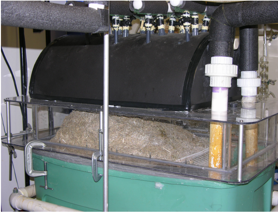
Figure 2-3. Photograph showing network of water sprayers on top of pile.
