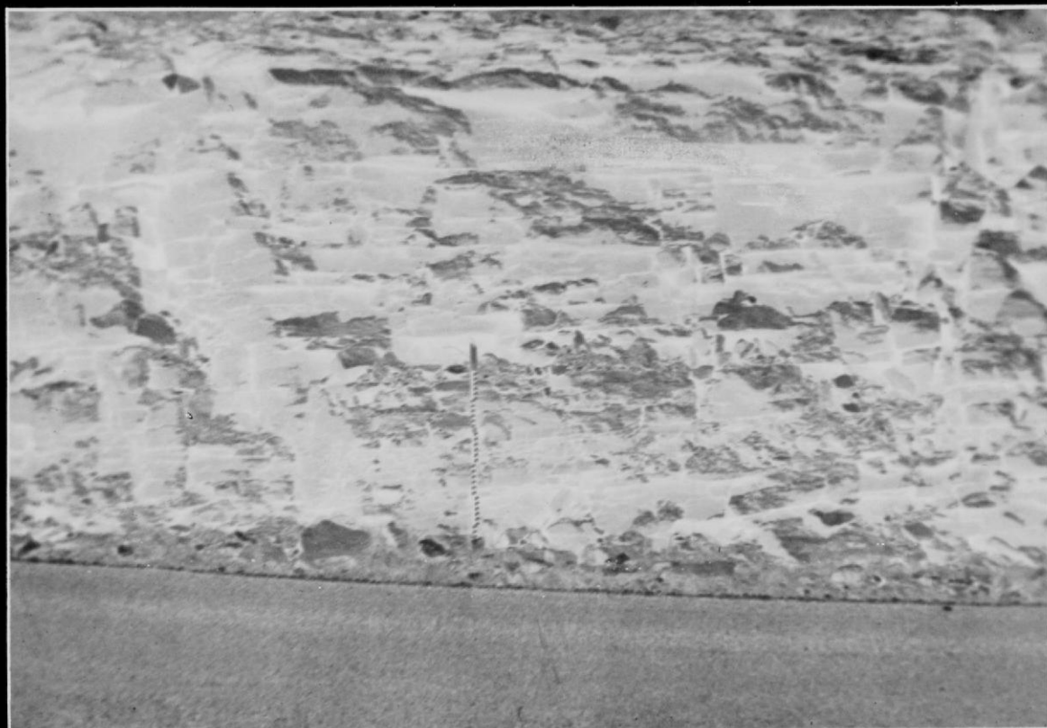
Cap Mountain Limestone Member in road cut where Ranch Road 501 cuts through the escarpment about two miles north of Pontotoc.
