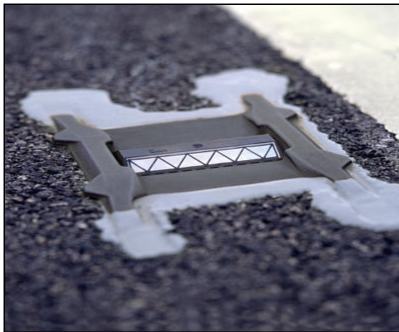
FIGURE 2 Typical snowplowable RRPM (7).
