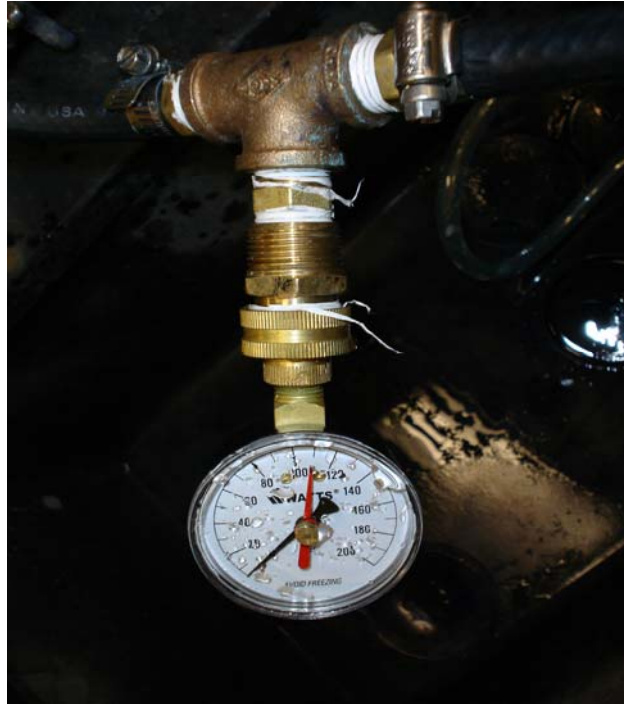
Figure 31: Hose pressure gauge connection.
