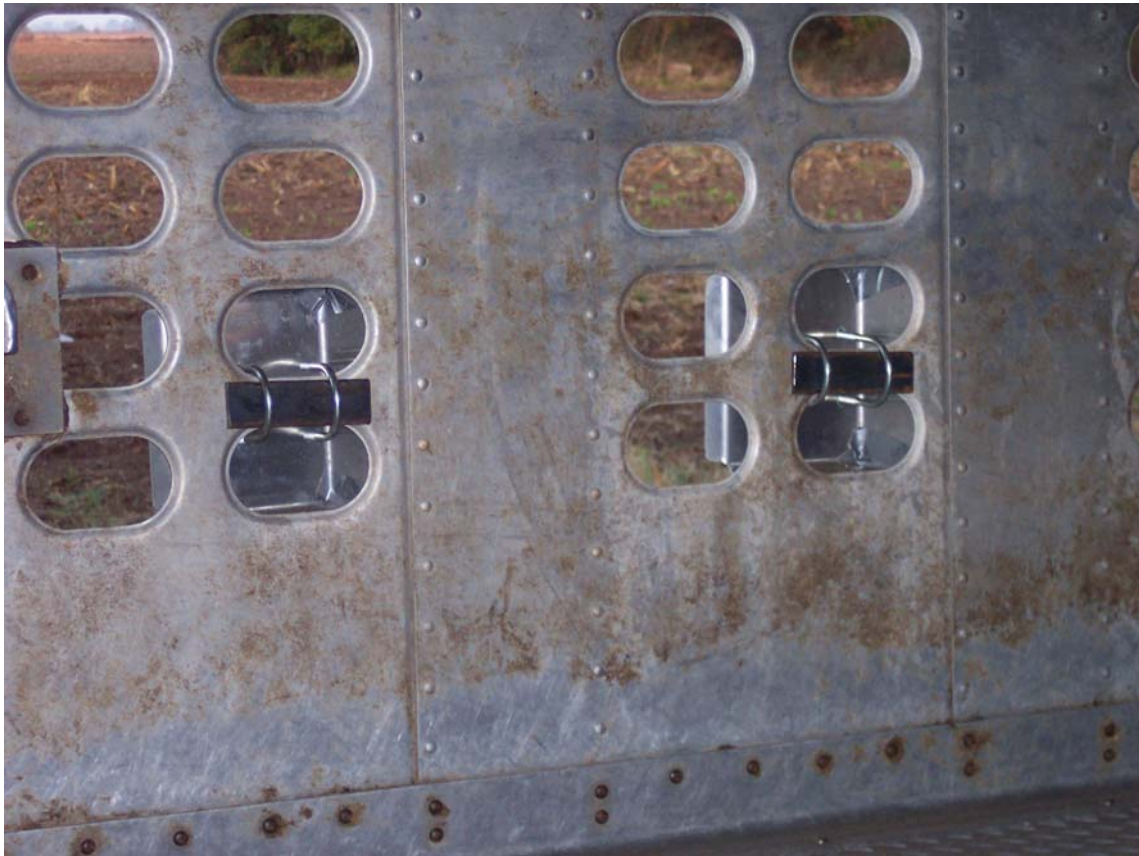
Figure 5. Steel plates used to distribute forces applied by scoops.
