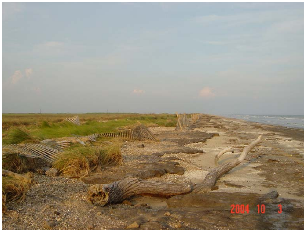
Fig. 1.2. The study area was damaged by tropical storm Ivan in 2004.
